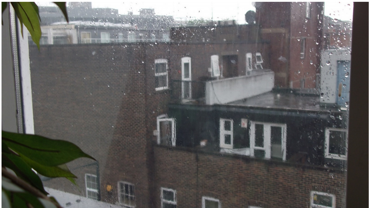
Mansard floor of 104/102 Euston Street and rear of 174/178 North Gower Street, showing escape gallery with the lift tower of 180 North Gower Street beyond, viewed from a 5 th floor office across Euston Street
