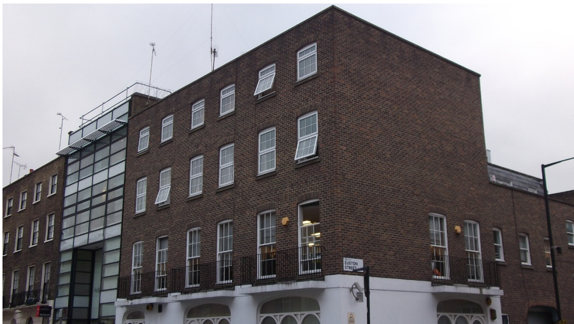
North east Corner of North Gower Street and Euston Street junction showing height difference between North Gower Street and Euston Street
