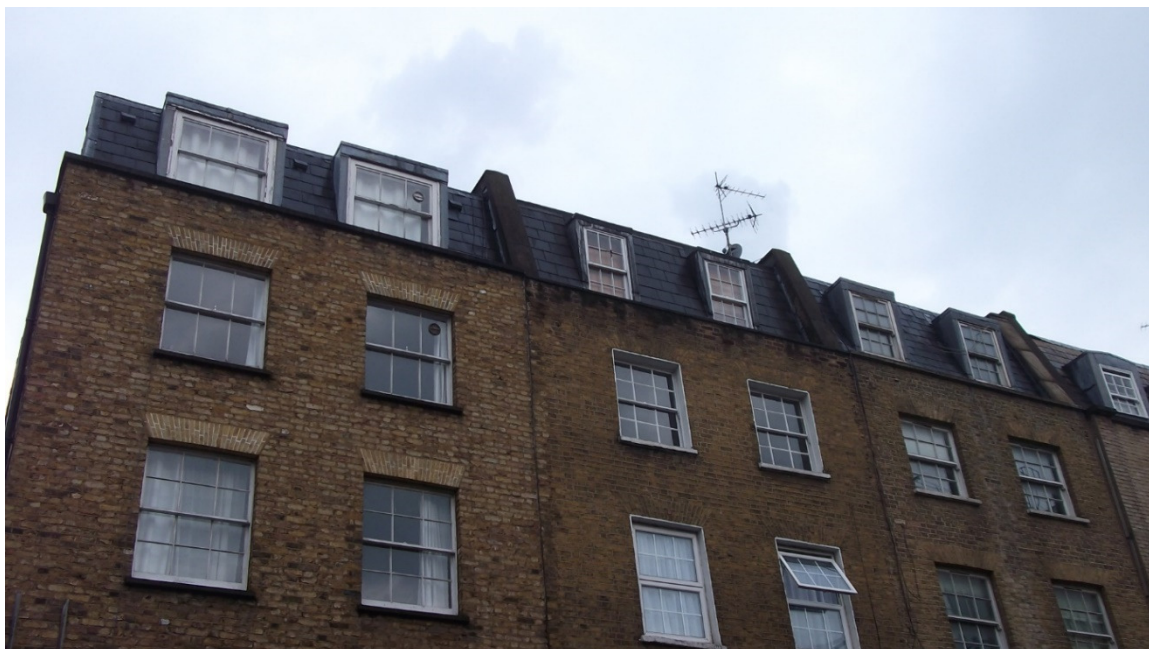
Detail of 172-166 North Gower Street showing existing mansard accommodation punctuated by dormers.
