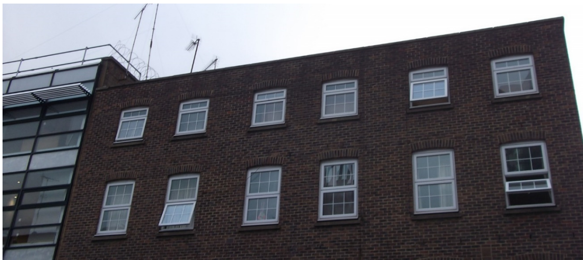
West elevation of 174-178 North Gower Street built c 1977-8 showing 180 North Gower Street, in modern style to left
