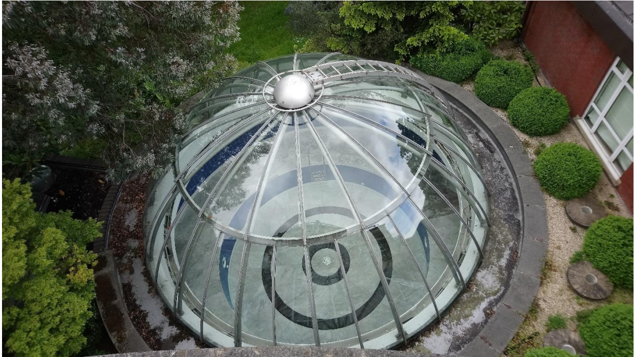
Figure 14. Pool seen from roof of the main house. Note close proximity of the new 1994 building to the pool and loss of the landscaped mound.
