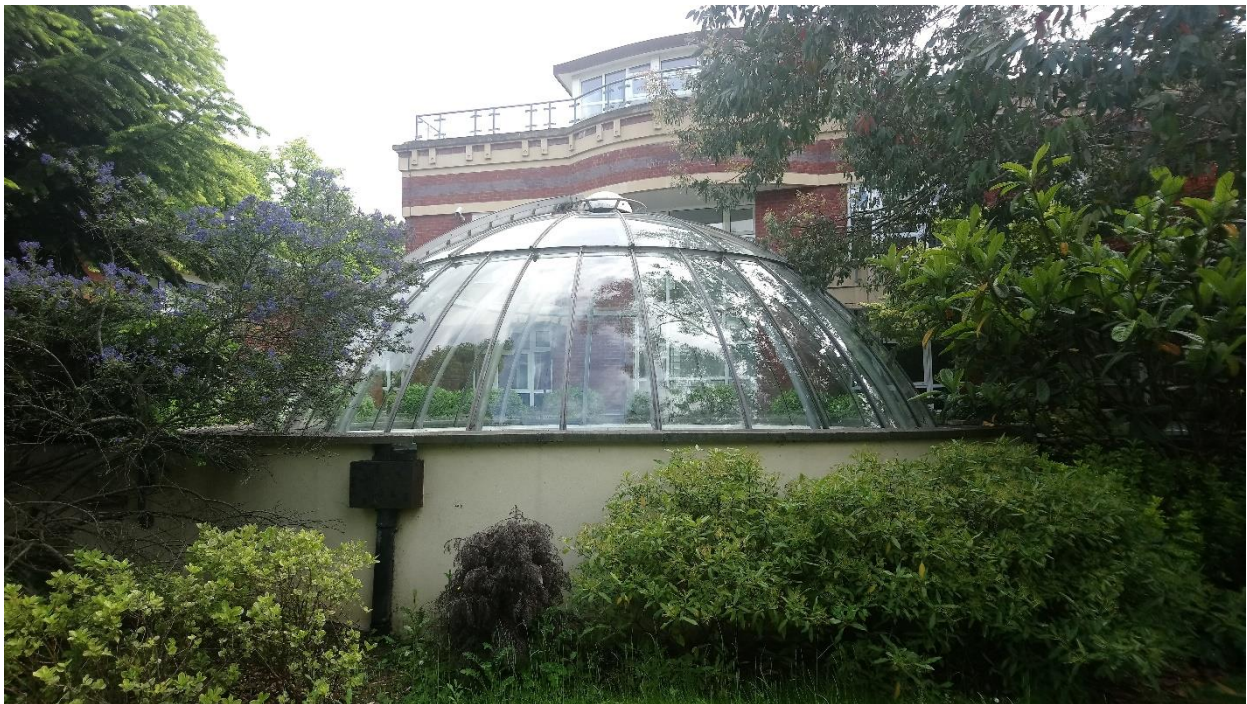
Figure 15. View of the pool from the garden. Note loss of the original landscaping which surrounded the pool and close proximity of the house to the east.
