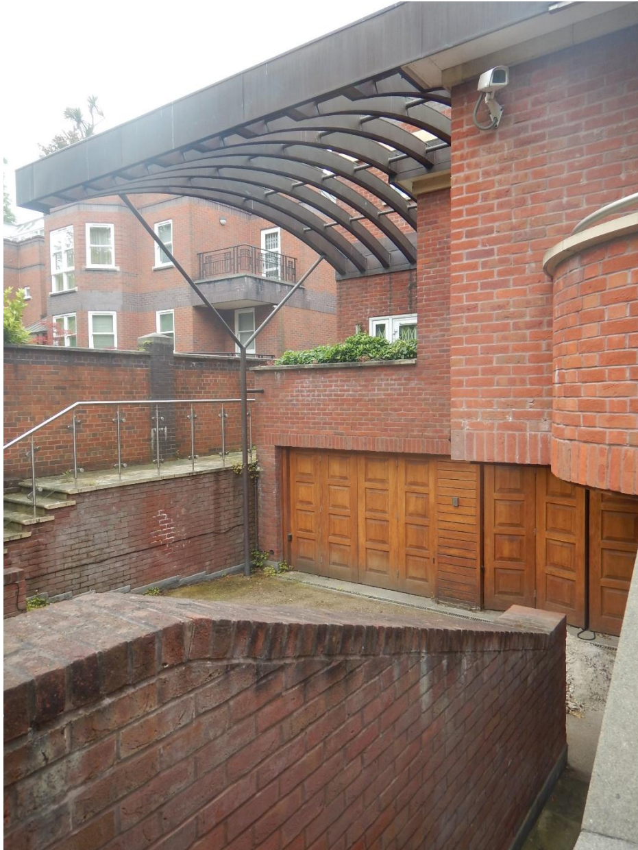
Figure 18. Main entrance of the house from Templewood Avenue. Note drop in level from the street and fragmentary nature of the façade contrasting with the formality of the main elevations and entranceways of houses seen elsewhere along the road.
