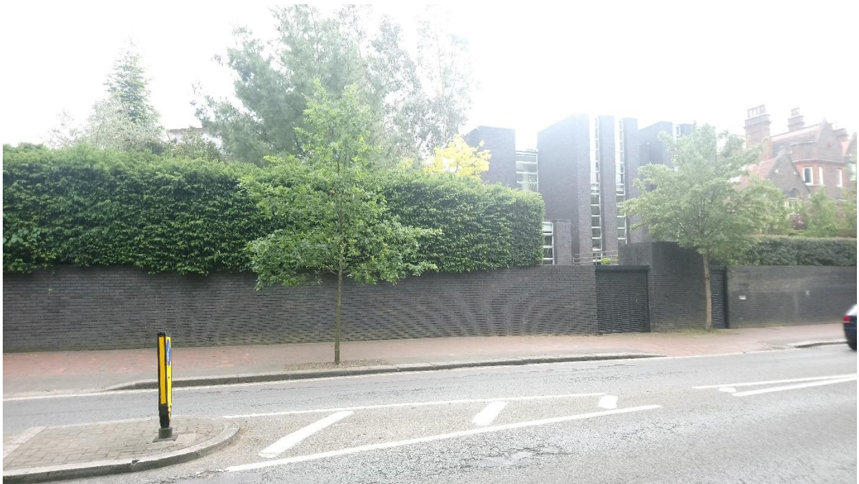
Figure 17. Schreiber House seen from the road to the north.
