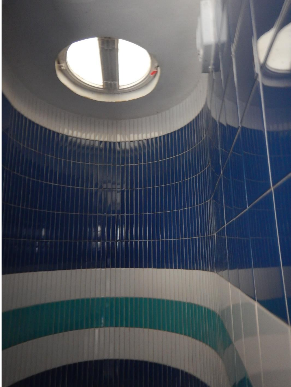
Figure 23. Roof of WC adjacent to the main pool.
