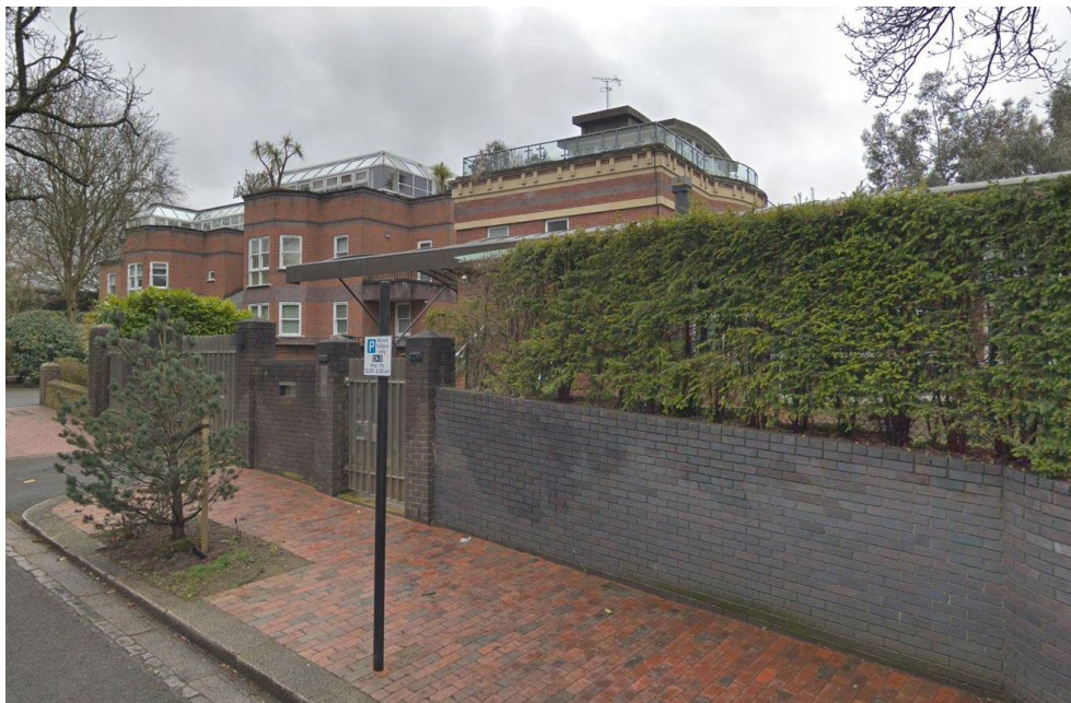
Figure 12. View of the site from Templewood Avenue. Note the development within the site converges with the building to the south.
