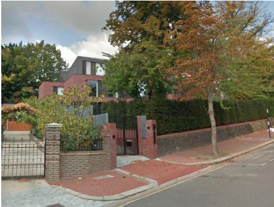
Figure 36. 17 Templewood Avenue as existing seen from the street.
