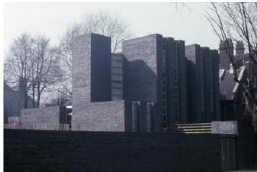
Figure 9. Early photograph of Schreiber House, taken from West Heath Road. Note dark stock blue 'engineering' brick.
