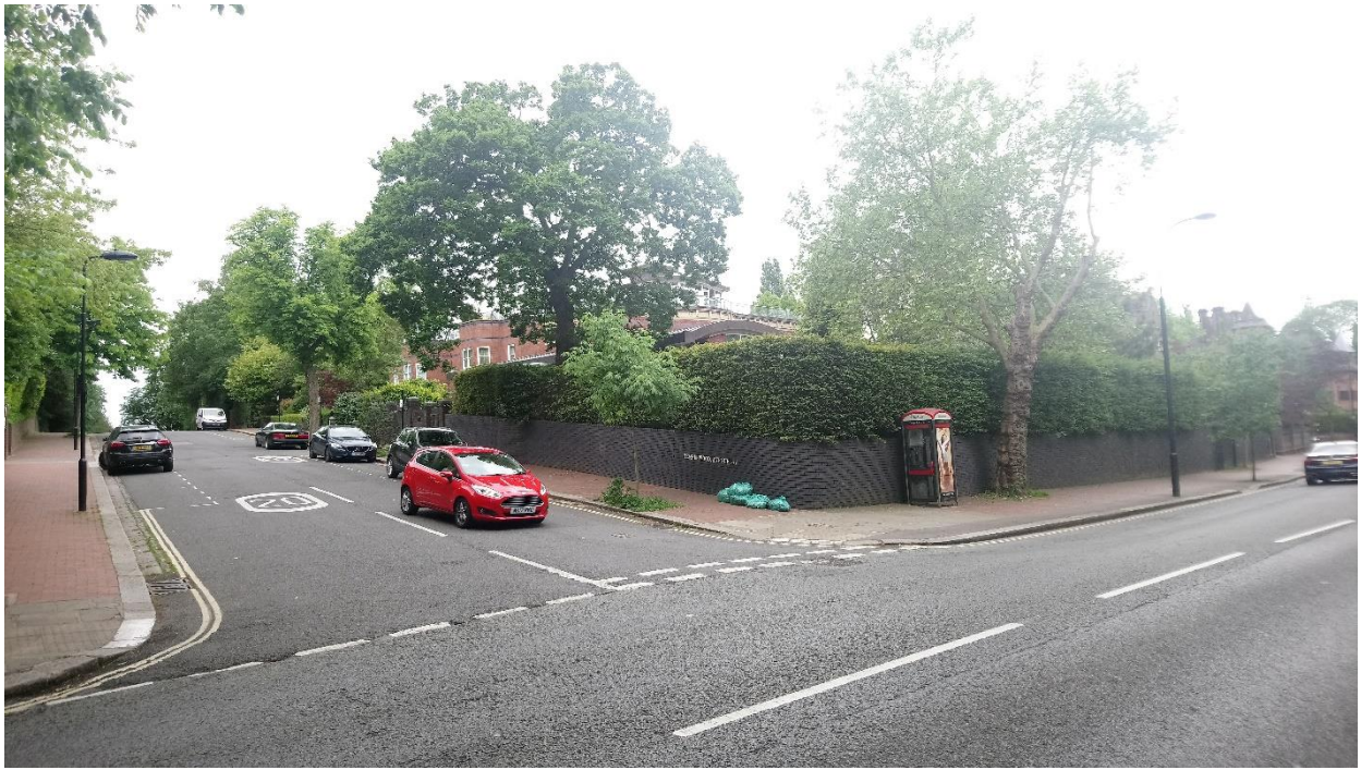
Figure 16. View of the site seen from the junction to the north. Note the dark engineering brick of the boundary wall indicating the extent of the original plot of Schreiber House.
