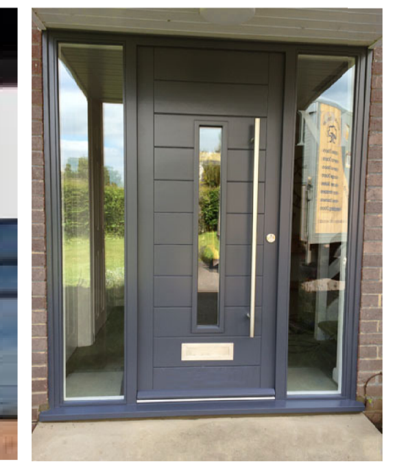
Key Ref No. 6. Dark coloured metal clad composite doors and windows
