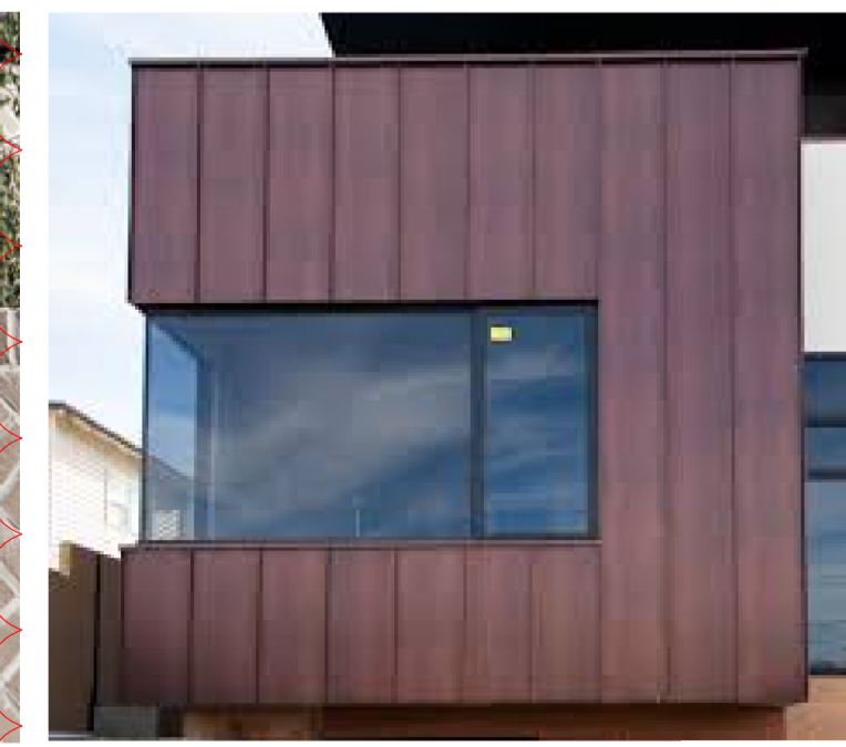
Key Ref No. 3. Pre-oxidised copper coloured standing seam cladding
