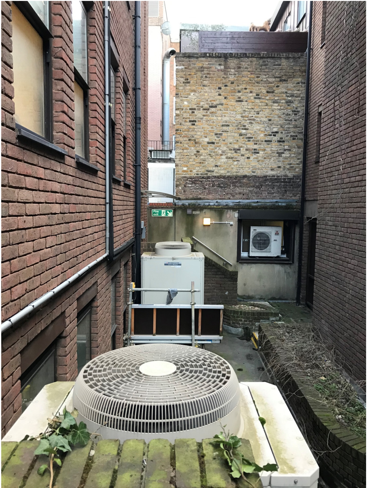
Photo E – Untreated Air Cooled Condensers behind 99 Grays Inn Road (Fanz House)
