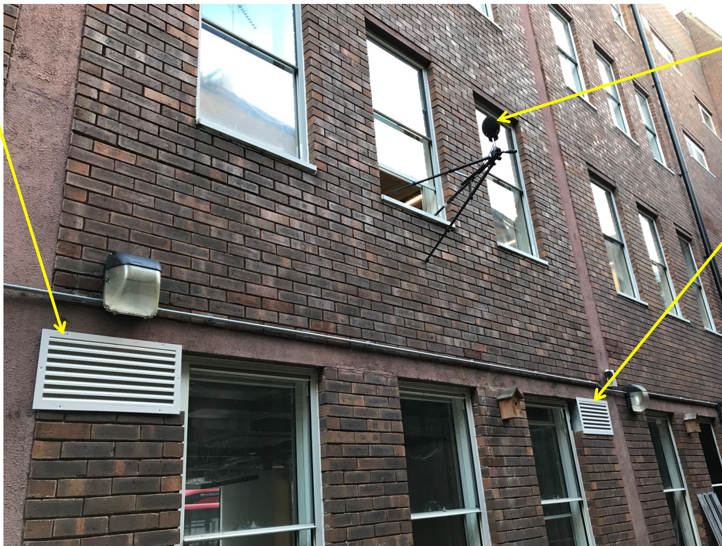
Photo C – Location of microphone above newly installed fresh air & exhaust louvres of ground floor heat recovery unit
