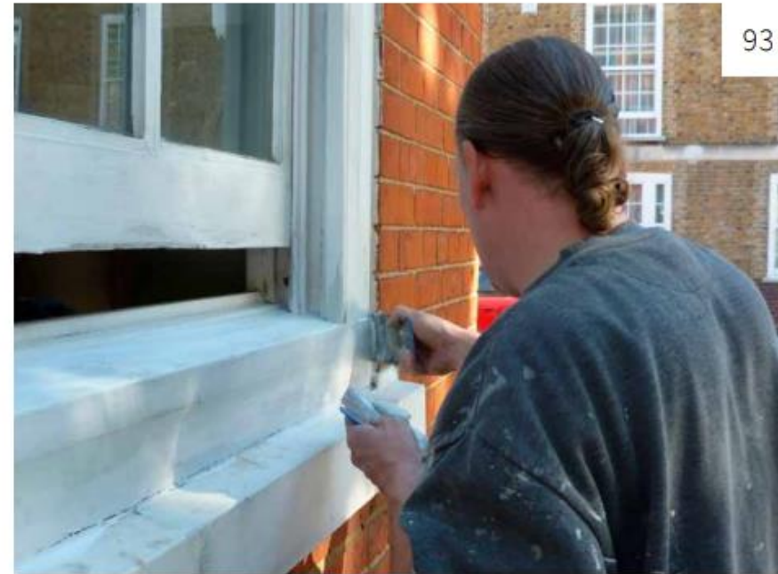
93. The decayed parts of the window being filled and primed ready for repainting.
