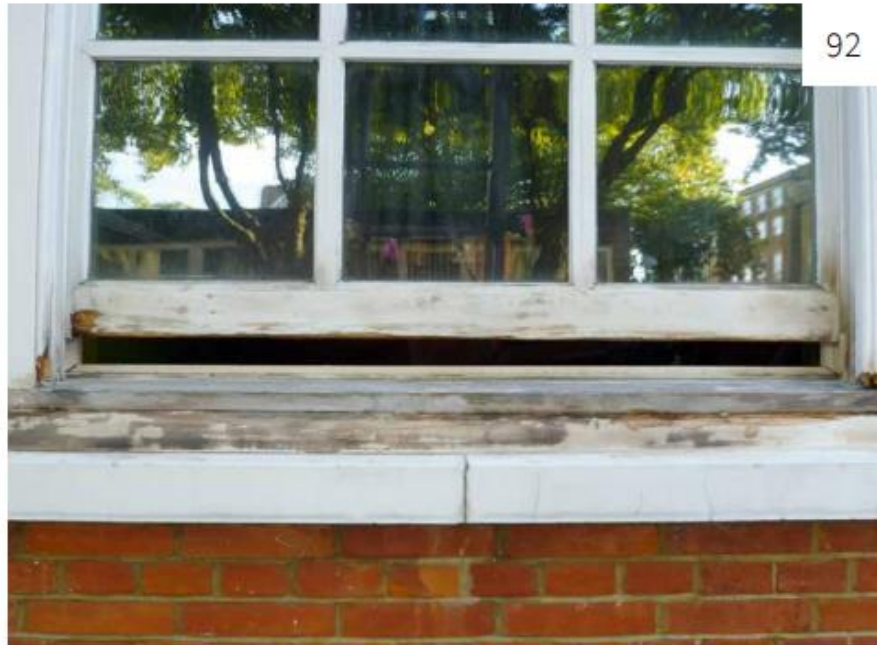
92. If paintwork is allowed to deteriorate on timber windows this can lead to decay of the timber as shown here to the lower more vulnerable parts of the window.
