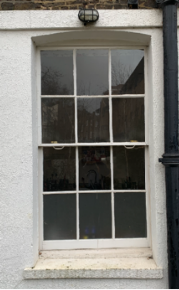
The existing sash window in the rear.
