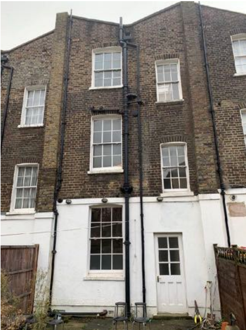
The rear elevation of the property
