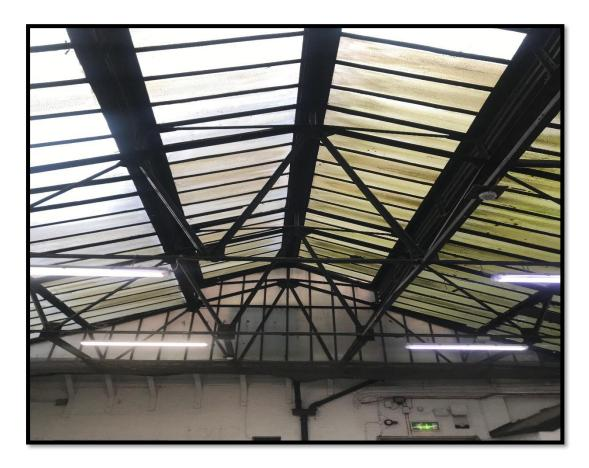
The glazing will be freed from the steel seating by hand using a combination of hand tools to prevent cracking/shattering of glass. The glazing panels will be lowered down to the floor by hand and placed into a waste skip.
