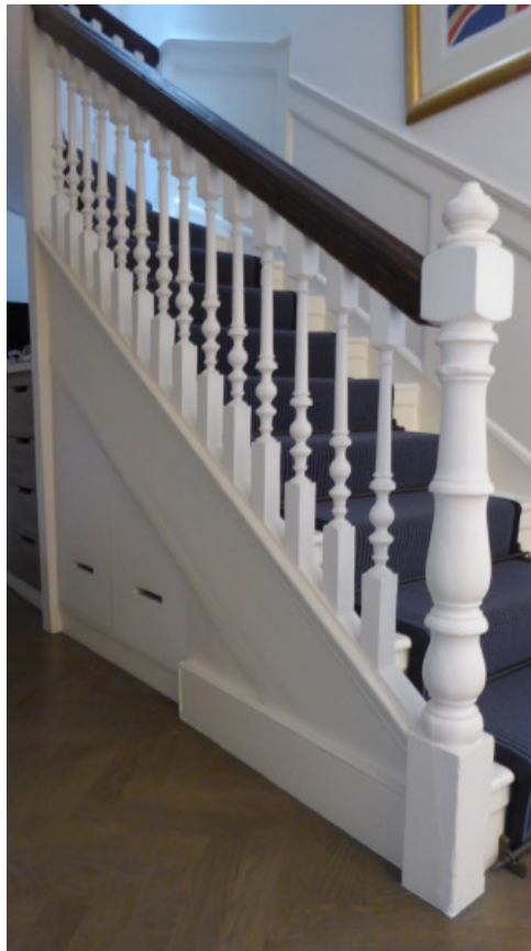
Existing stairs (first to top floor)
