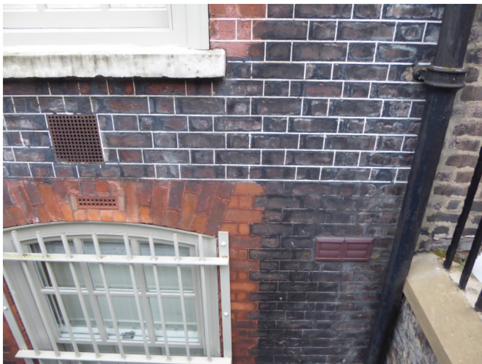
Existing ventilation grilles
