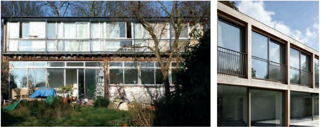
Figure 4: 3 The Hexagon Rear Facade prior and post works in 2012
