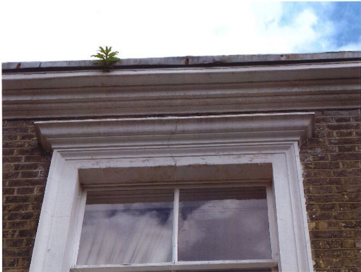
DAMPNESS AFFECTING TOP OF FRONT MAIN WALL.
