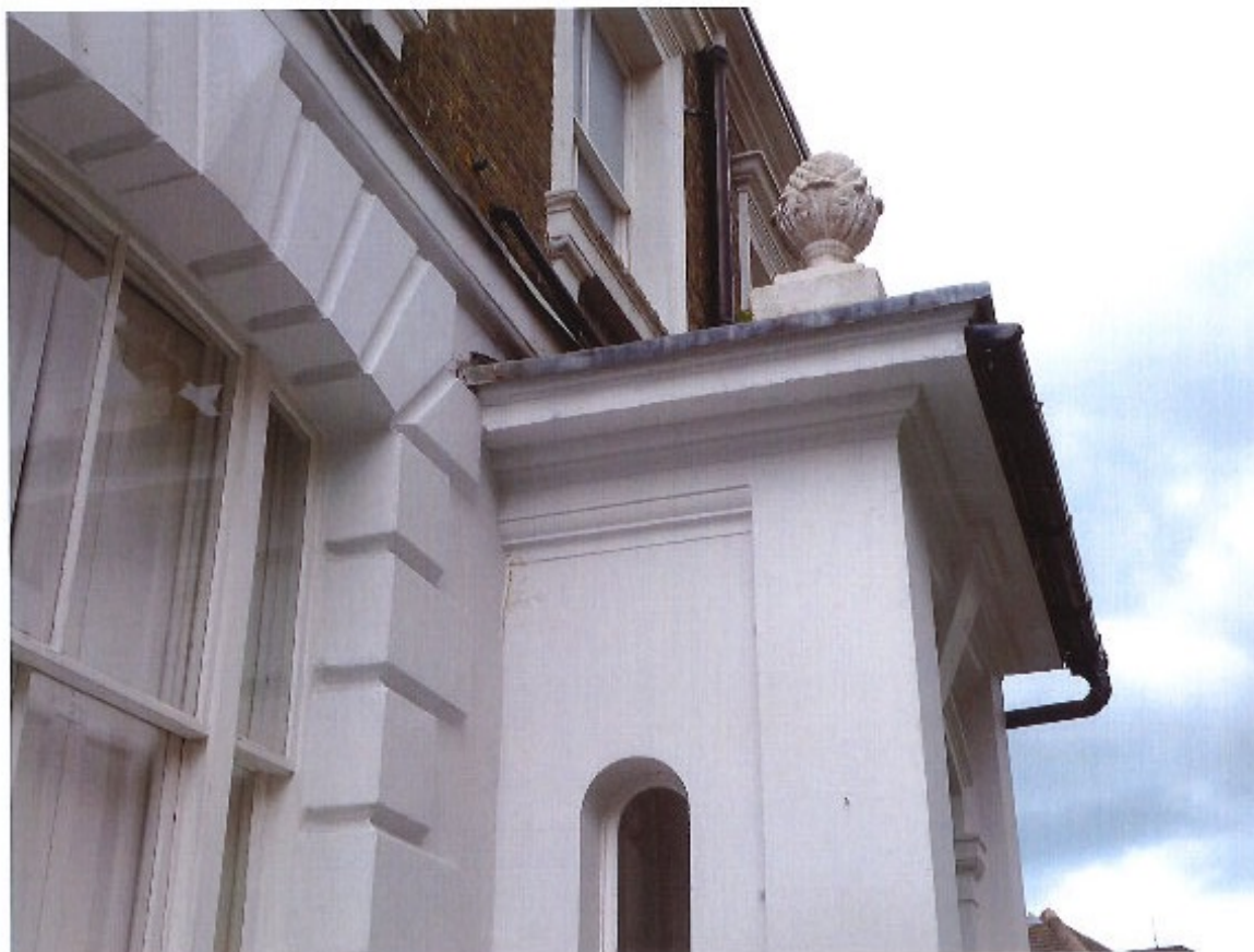
DAMPNESS AFFECTING LEFT SIDE OF PORTICO STRUCTURE
