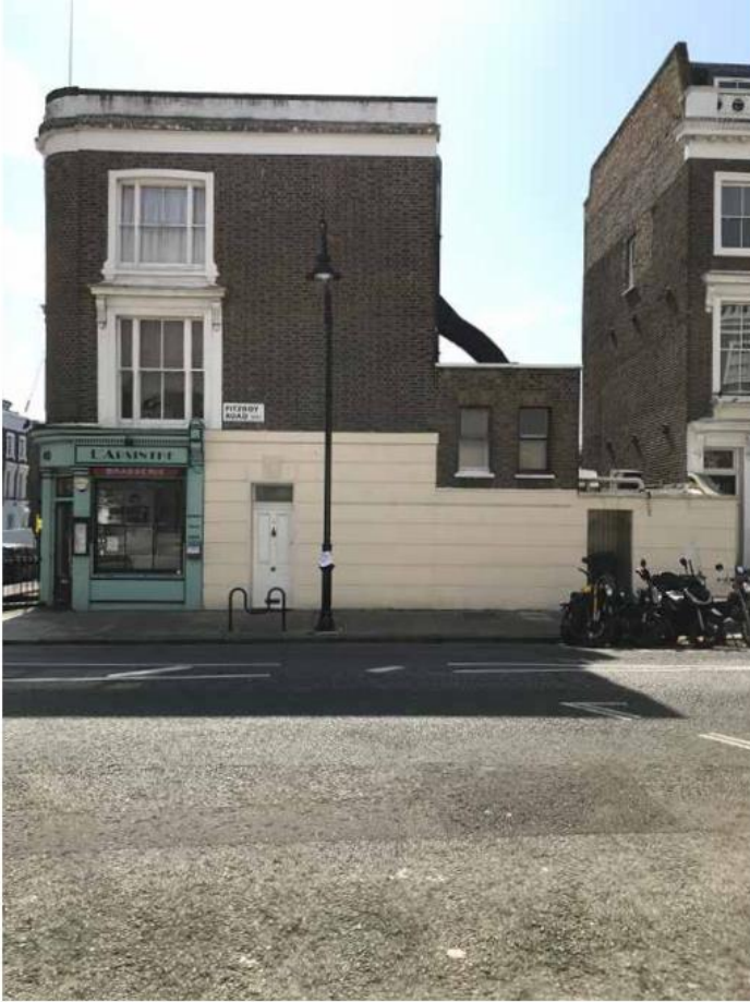
Existing frontage to Fitzroy Road
