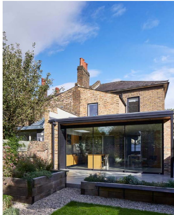
Notch House, Hackney
