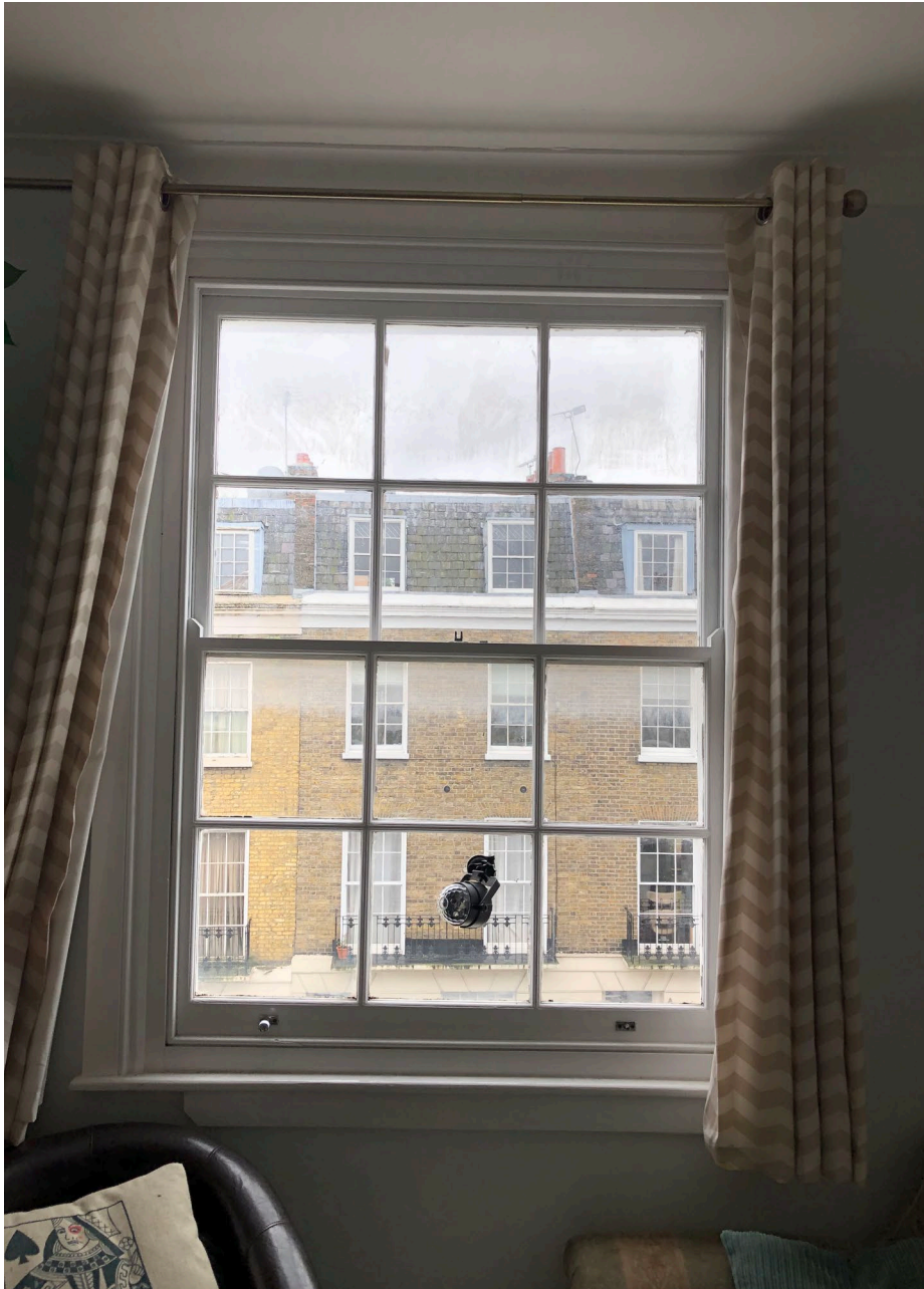
Figure 9: Internal view of window at second floor level - Lounge (Flat C)
