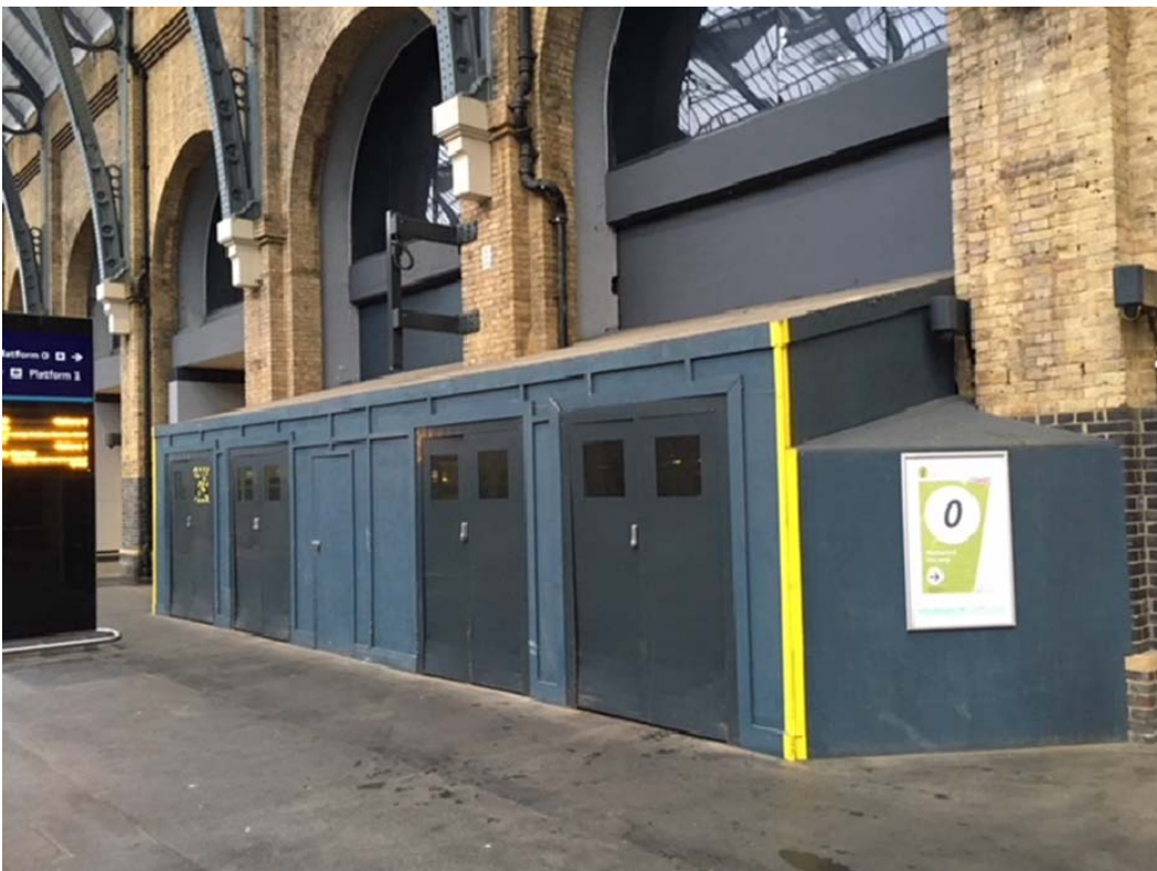
(Figure 1- Photograph of existing store platform 1 to be removed)
