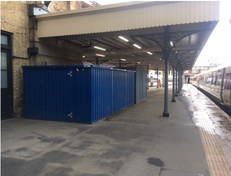
(Figure 2- Photograph of existing store platform 8 to be removed)
