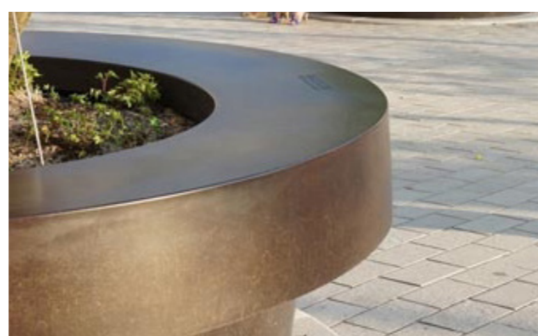
Bronze effect steel to all metalwork such as armrests, bicycle stands, lighting columns and litter bins.
