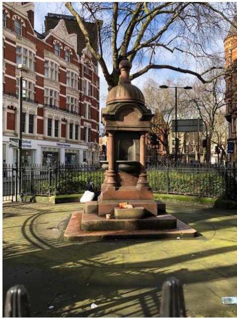
Figure 2: The grade II listed drinking fountain.
