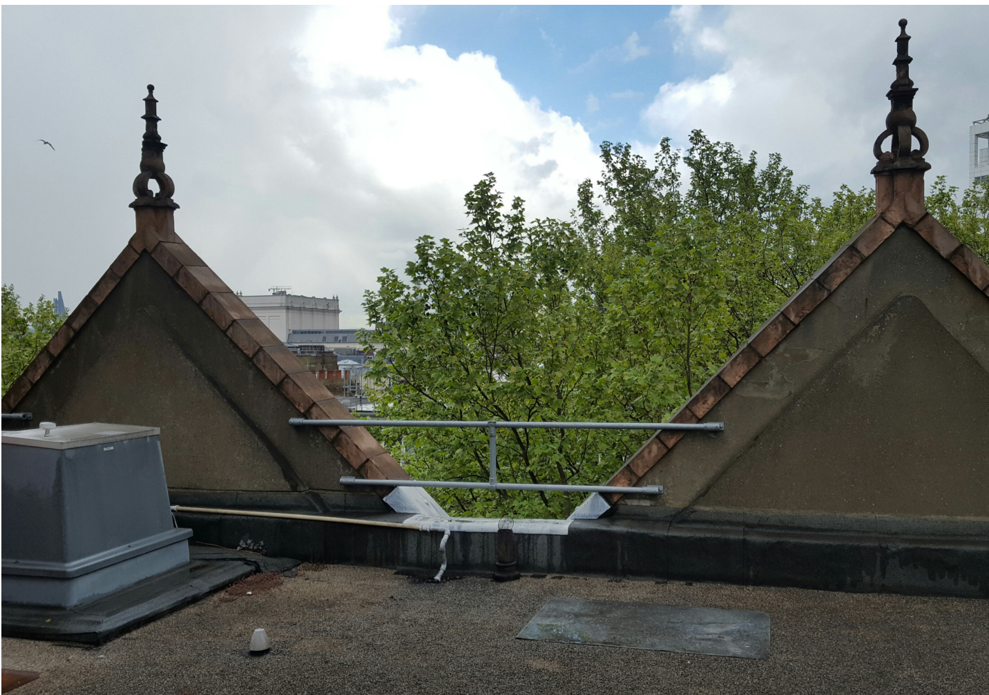
Existing roof gables on Shaftesbury Avenue elevation showing line of original pitched roof
