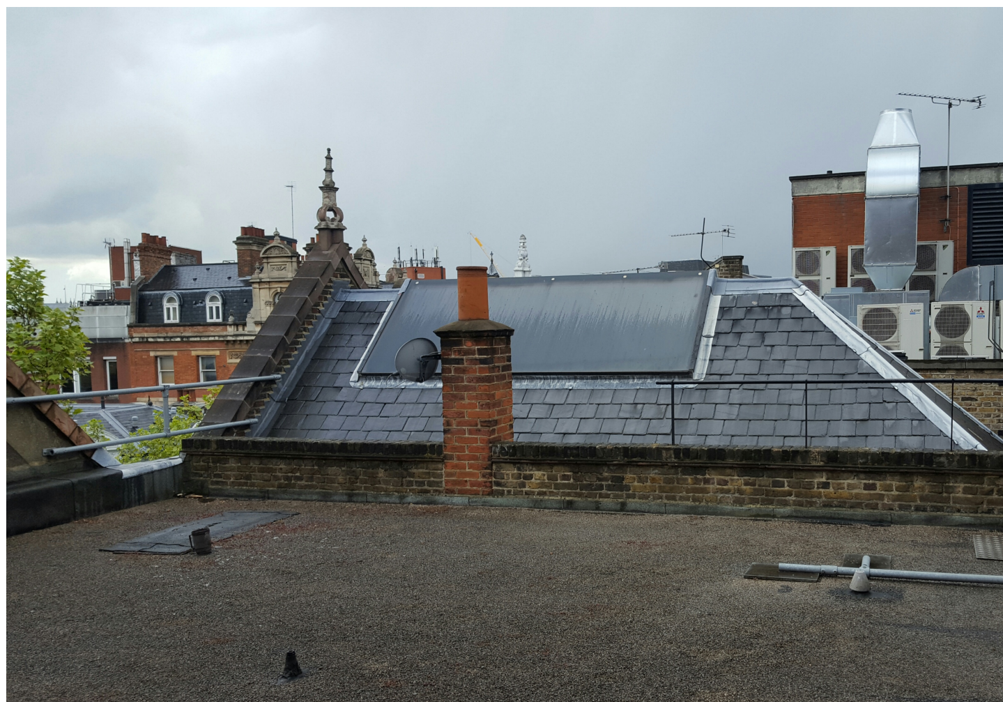
Adjacent pitched roof at 117 Shaftesbury Avenue
