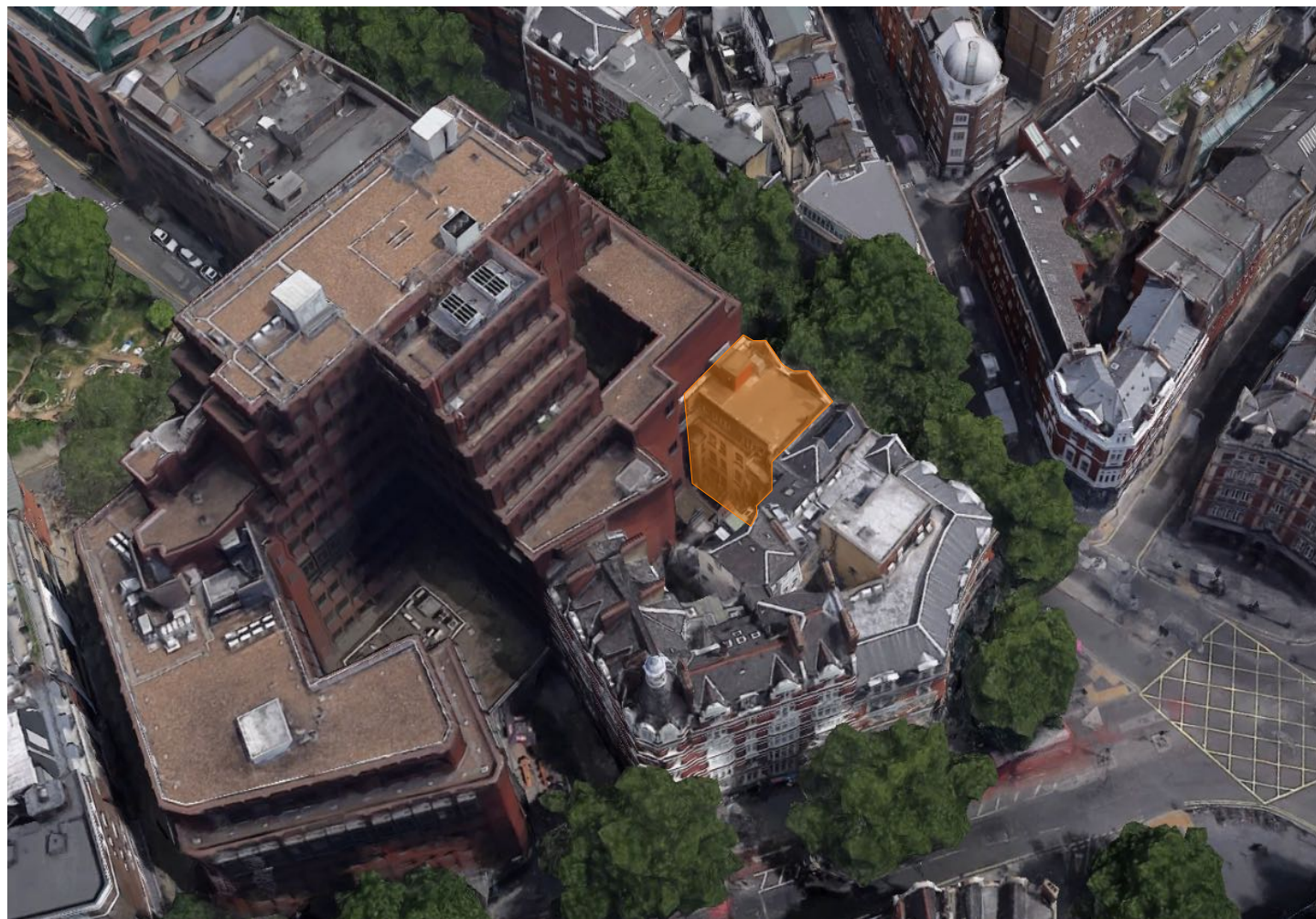
4. Aerial view from rear of 119 Shaftesbury Avenue
