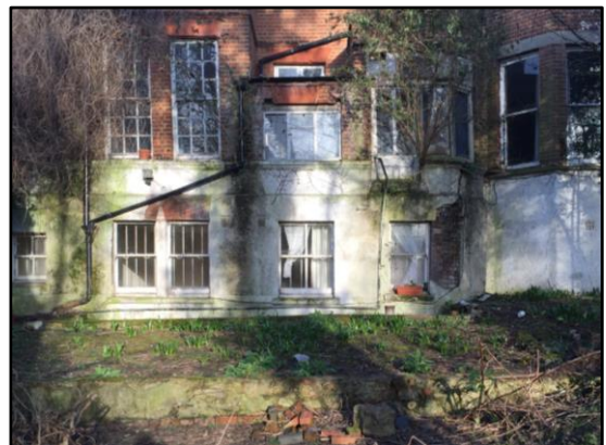
Figure 2.7: Lower Ground Floor Level to Rear of Elm Tree House
