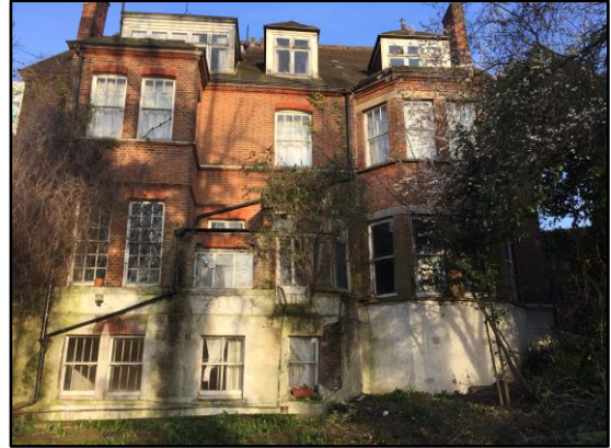
Figure 2.3: Rear of Elm Tree House
