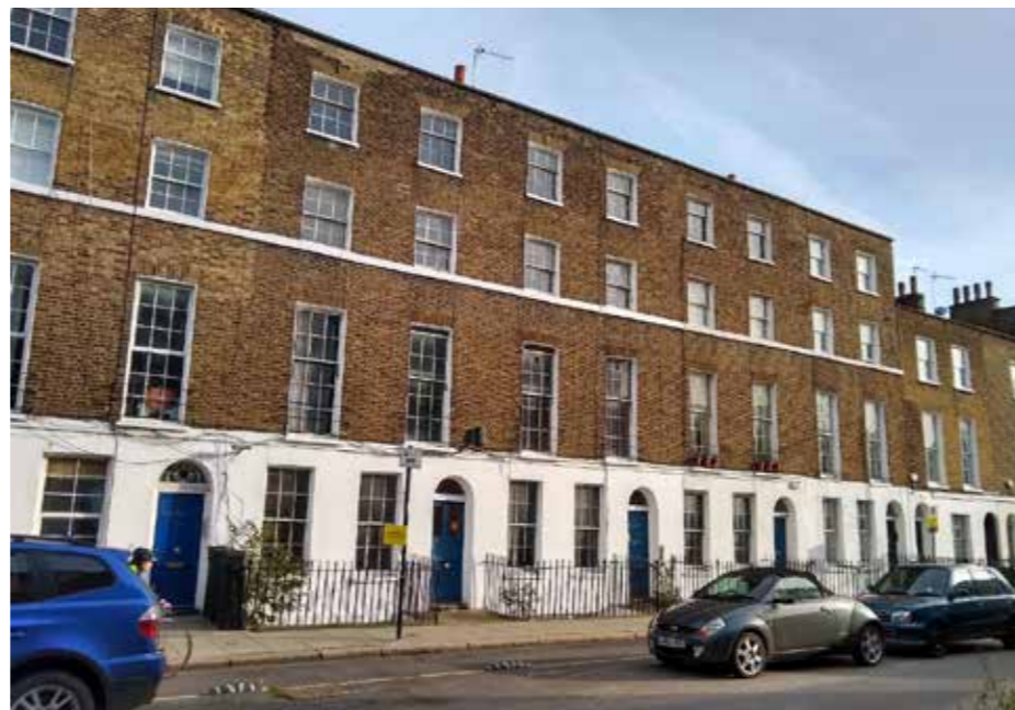
Figure 5.3 listed buildings to the south of the Site along Royal College Street
