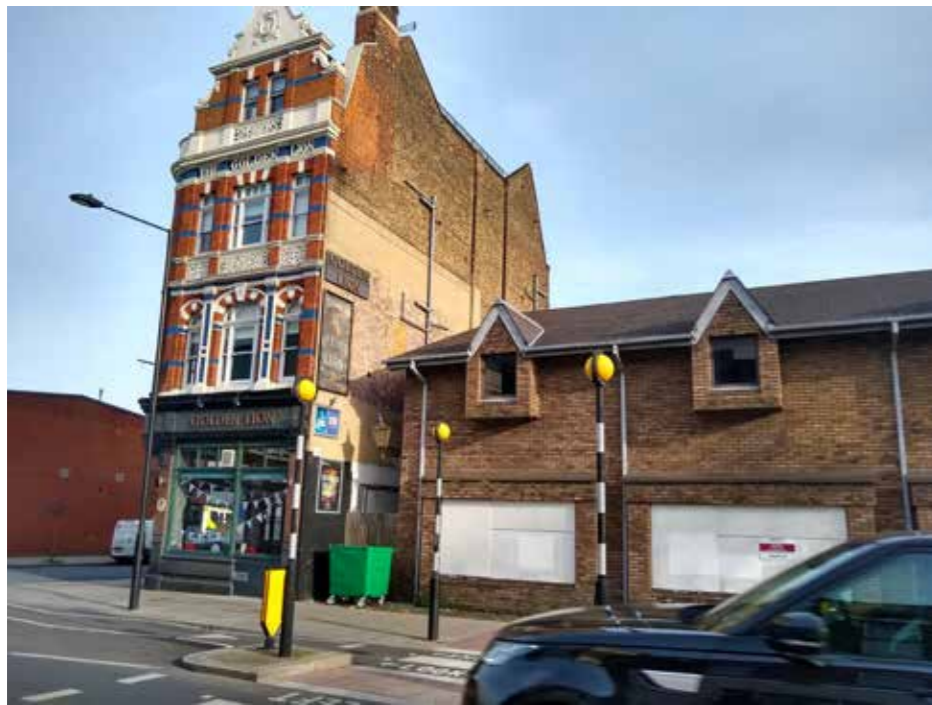
Figure 5.5 The Golden Lion Public House and adjacent Site buildings
