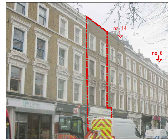
5. STREETSCENE PERSPECTIVE DEMONSTRATING NEIGHBORING ROOF EXTENSIONS AND ROOF TERRACES AT NO. 6 & 14. NO.6 ROOF TERRACE IS NOT VISIBLE AS IT IS SET BACK.
