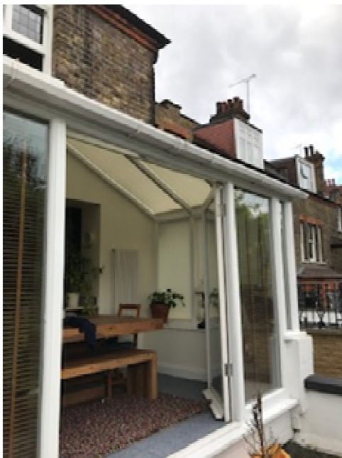
4. Rear elevation of the existing conservatory
