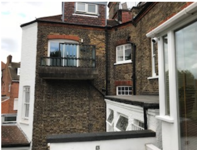
6. Views of the windows in the rear elevation and side elevation of the three storey rear extension at the neighbouring properties at no. 39 from the rear of the existing conservatory
