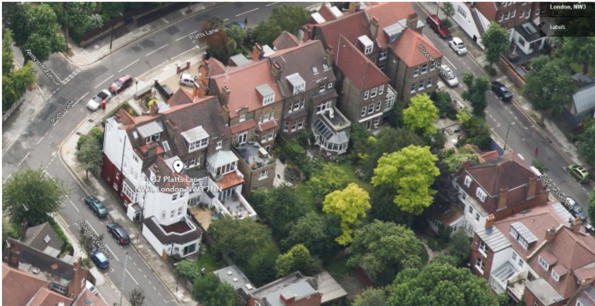
1. Ariel view of the rear of properties along Platt's Lane
