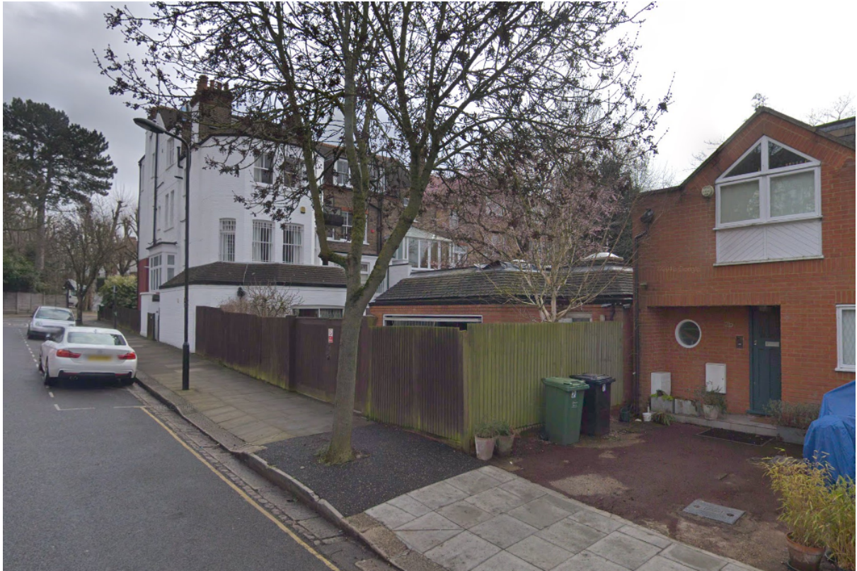
9. View of the existing conservatory from Briardale Gardens looking south.
