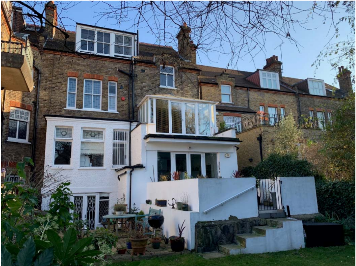
3. Rear elevation of building showing the existing conservatory
