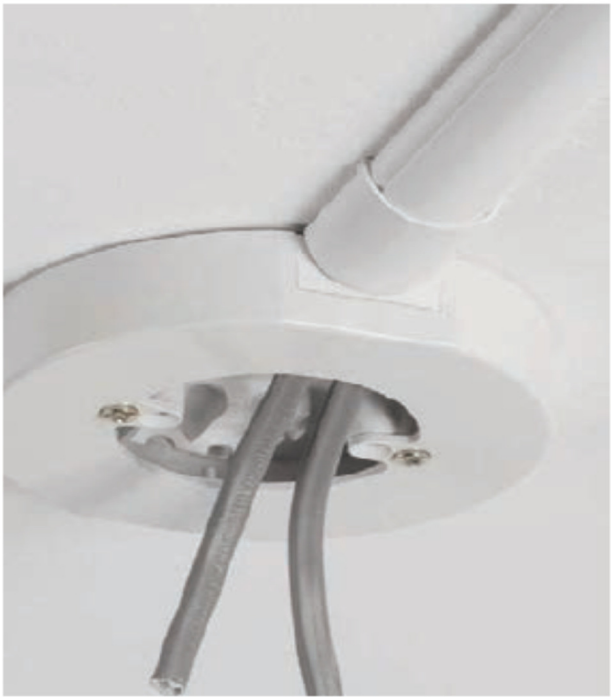
Termination of the trunking to ceiling rose with purpose designed accessory
