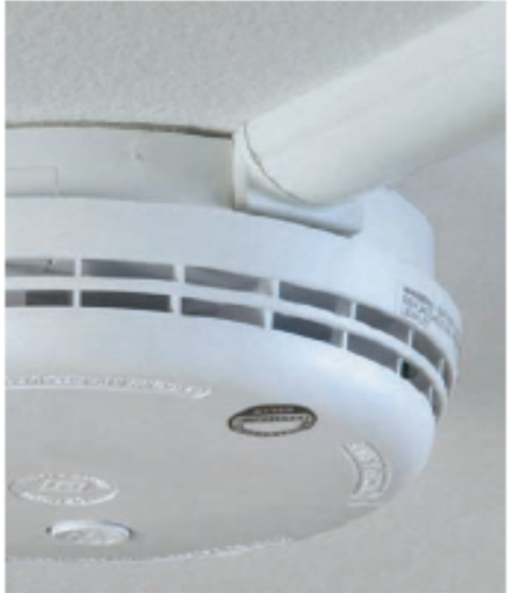
Purpose designed circular adaptor for smoke detectors.
