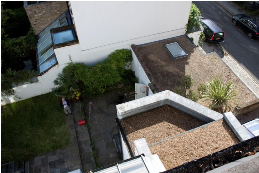
A. Existing garage roof
