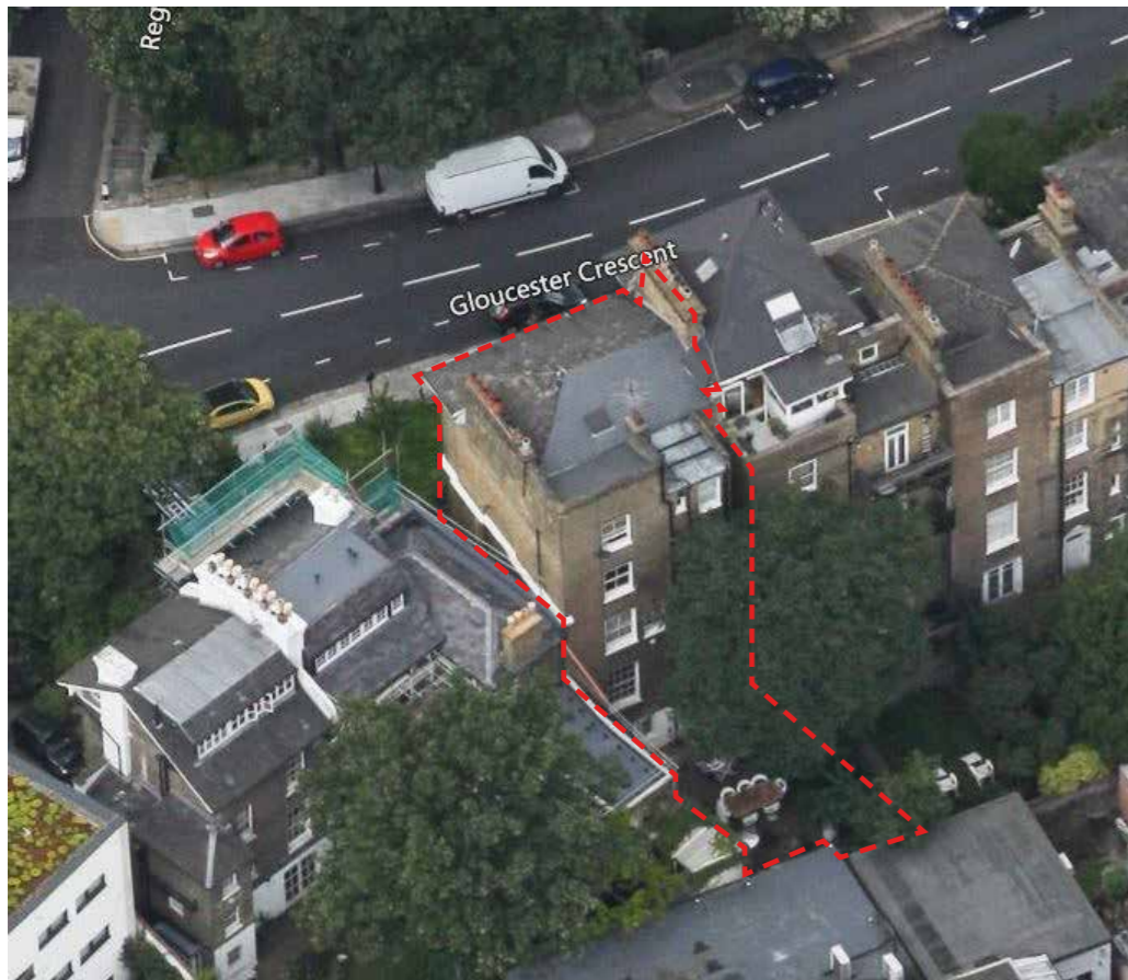
Bing map 3d views showing the front and rear of the property
