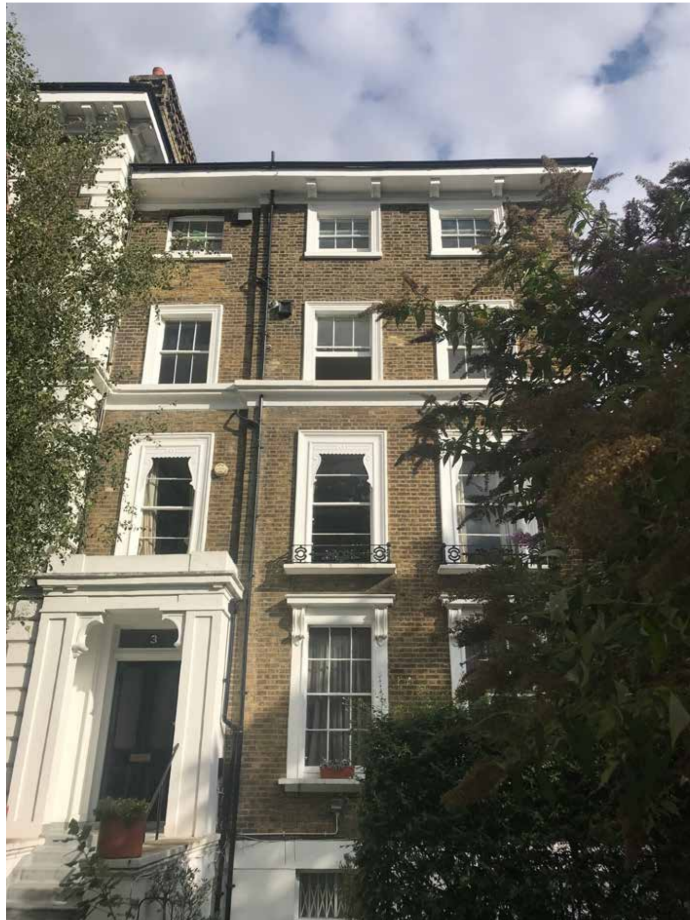
View of the front of 3 Gloucester Crescent. There is no specific listing information pertaining to the internal condition of the property. Flat 4 is the dwelling on the second floor of the property.
