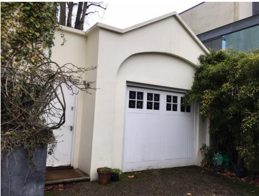
2 Existing side garage extension – to be demolished
