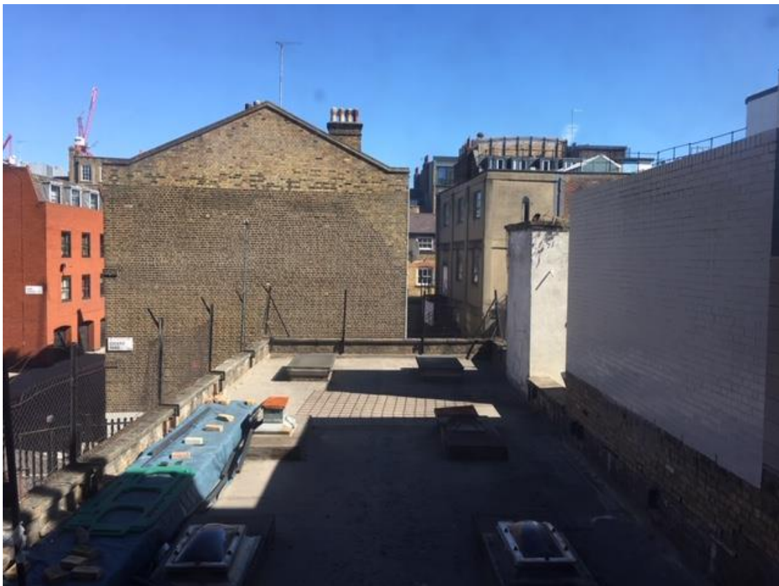
4. Roof top above no.15 ground floor extension
