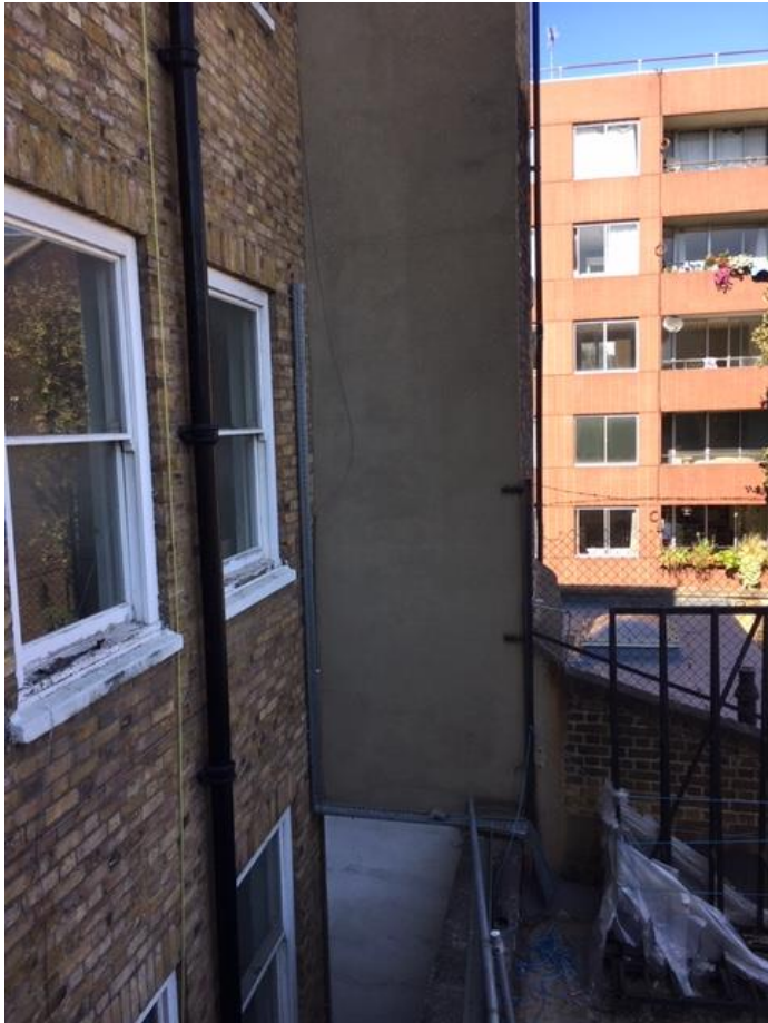
5. Rear face of no. 15 looking north towards no. 16 and Northington Street
