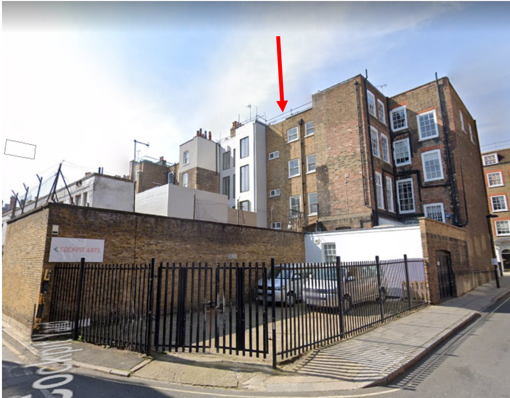
3. Rear view (arrow to no. 15)
