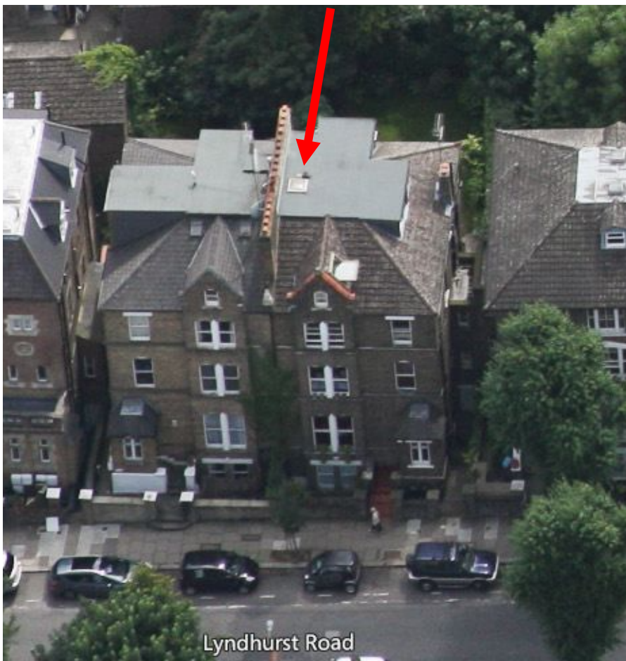
2. Aerial image showing existing rooflight
