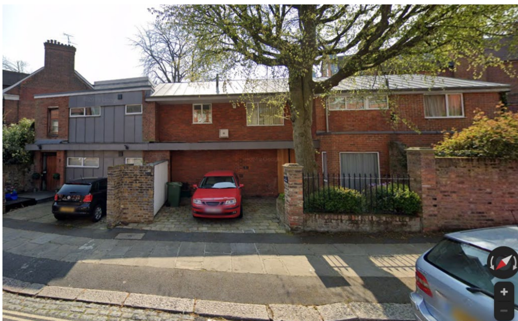
Current street view: 4A is the red brick house centre and right, with the sloping roof, 4B is the small metal clad structure to the left, clearly subordinate in size and visually to 4A. (Image source: Google street view (accessed Feb 10, 2020))
