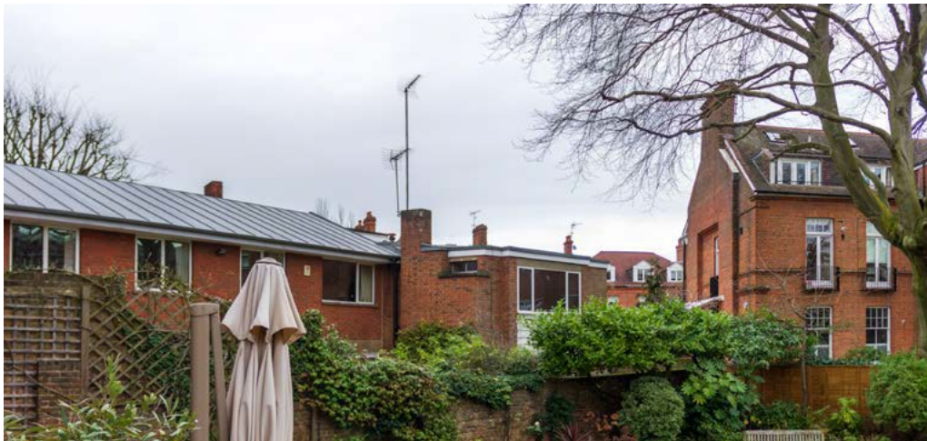
The existing building
