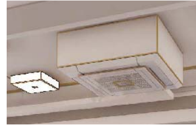
CEILING CASSETTE (In plywood boxing. See Dwg. M&E-P02 for detail).
