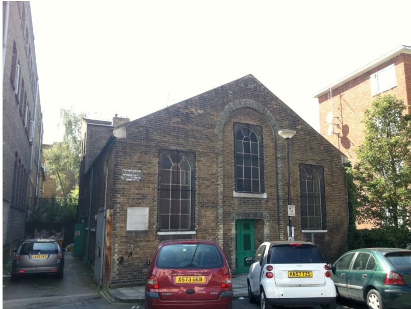
Photo No. 1 Front Elevation.
