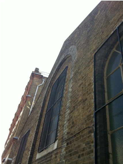
Photo No. 5 Front Elevation Detail.
