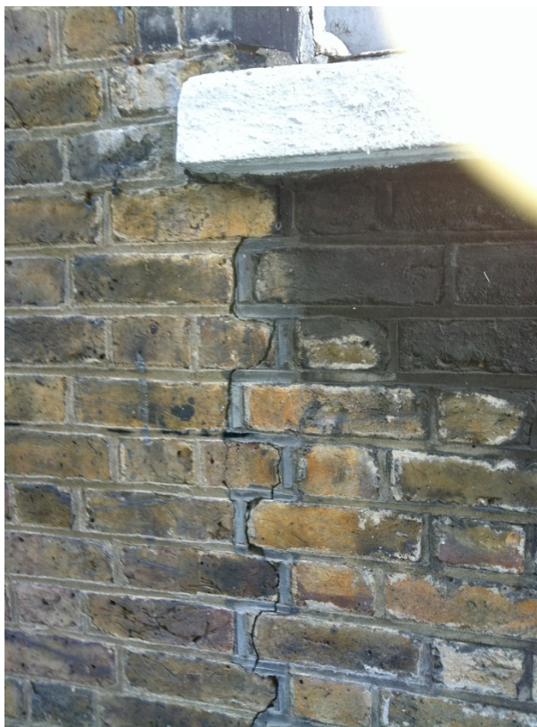
Photo No. 11 Repaired crack in flank wall apron adjacent to front wall.
