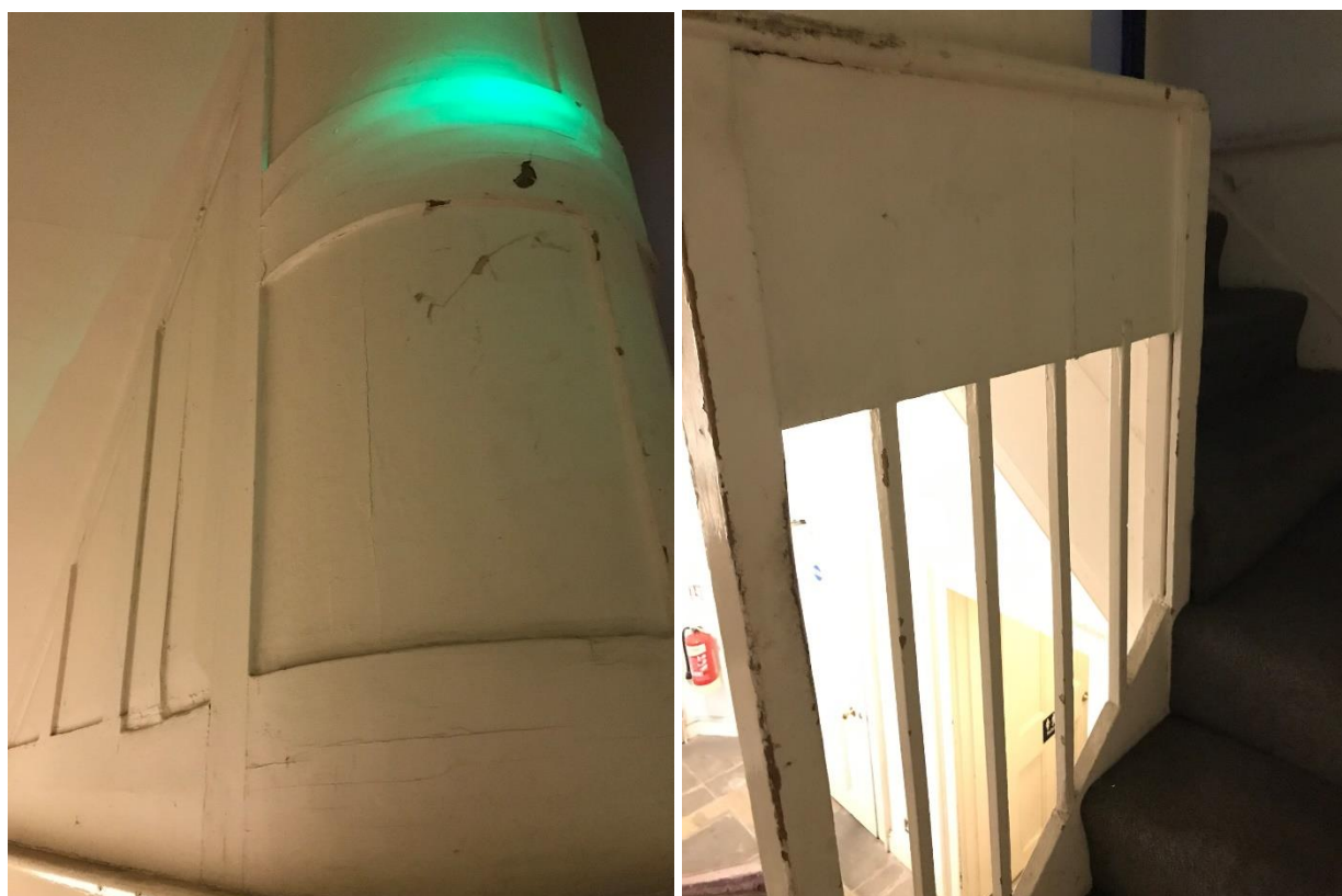
Figure 26 Rail and style timber panelling in the staircase between ground and basement levels.
