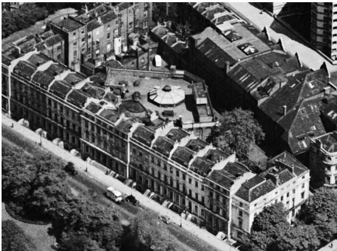
Figure 4 Aerial photograph from the south-west, 1946. Whilst most houses in the terrace have M-shaped roofs with the front in mansard form, the central three buildings and the end pavilions have full height attic storeys with pitched roof behind. The rear part of the roofs of nos. 17 and 19 is restricted by the Diorama's conical rooflight. Britain From Above, ref: EAW000542.
