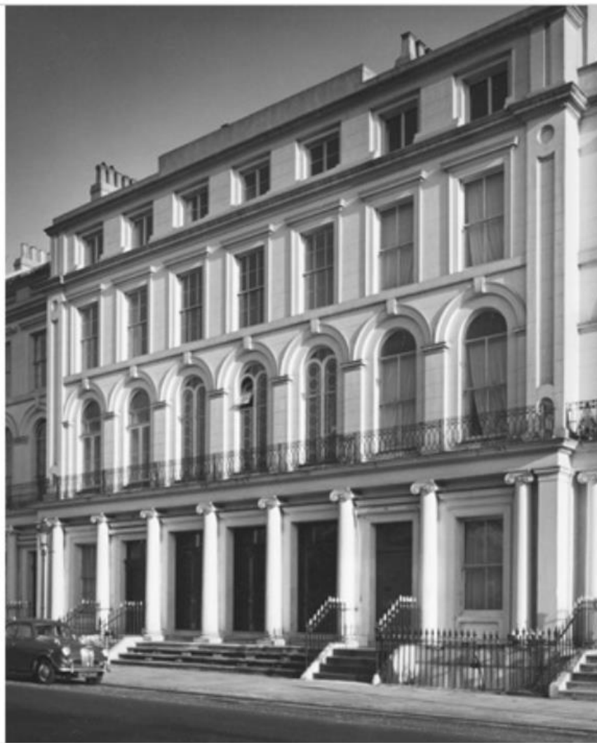
Figure 5 1962 photograph of the front elevation of 17-19 Park Square East. The 1850s chapel conversion of no. 18 included the removal of the original ground floor windows to create three doorways. RIBA Pix ref no.: RIBA5342.
