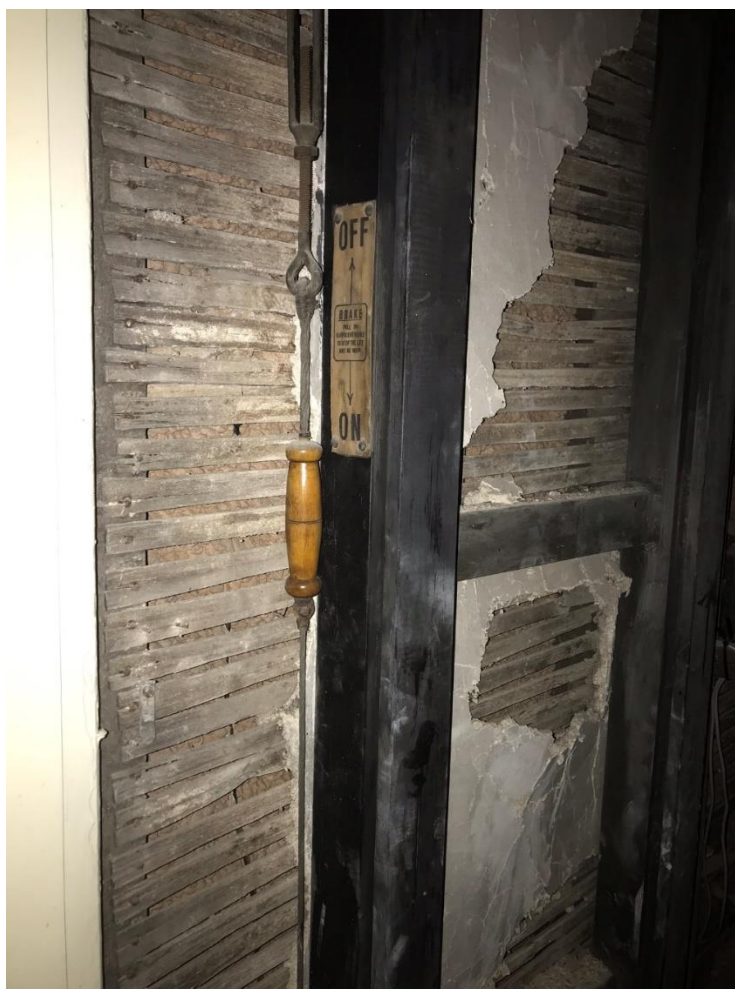
Figure 27 Lath and plaster internal wall within the first floor cupboard. There is a pulley system fixed to the internal walls at ground, basement and first floor.
