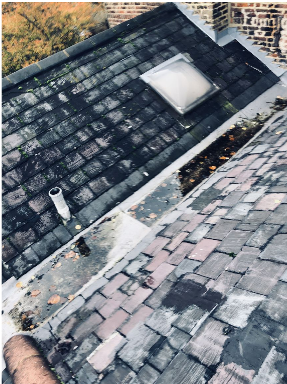
View of Valley Gutter and abutment Flashings
