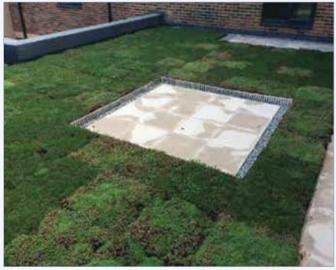
The modular sections mean detailing around objects is a simple process and clean lines are created. Hard landscaping sections such as paving and decking, mounted onto Wallbarn pedestals, can be added to the area to allow for regular access. As everything is suspended on top of the deck, drainage is uninterrupted.
