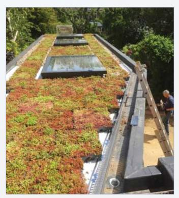
The edges should be filled with a border of washed riverstones, in accordance with the GRO code of practice. Objects such as roof lights and cables should be surrounded with riverstones to prevent root invasion and act as a fire break.
