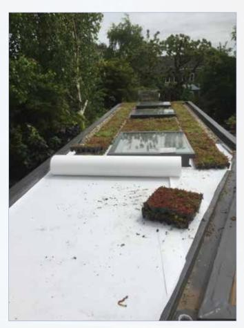
A separation and filtration geotexile layer should be firstly installed onto the deck. This protects the waterproofing and prevents abrasive damage. Wallbarn can supply a 300gsm recycled fleece for this purpose.
