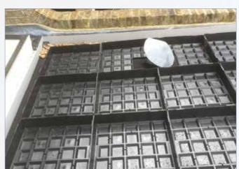
The module measures 500 x 500 x 100mm. As four units make up exactly one square metre estimating is a far easier process.
