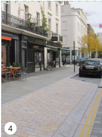
4 Tricolour granite pad at pavement level
