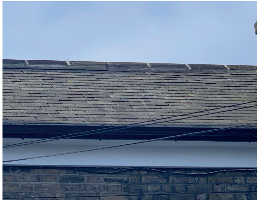
Above: Front Elevation_ Re-usable existing tiles
