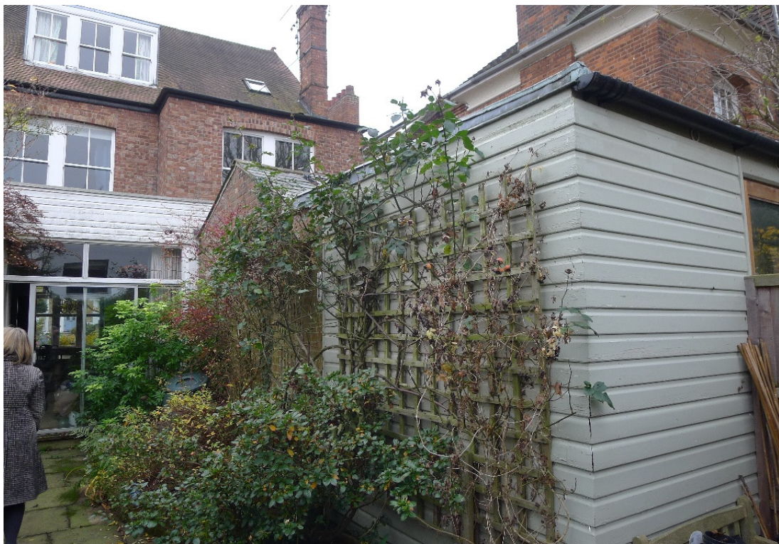
Rear elevation and studio extension showing original offshoot with pitched roof.
