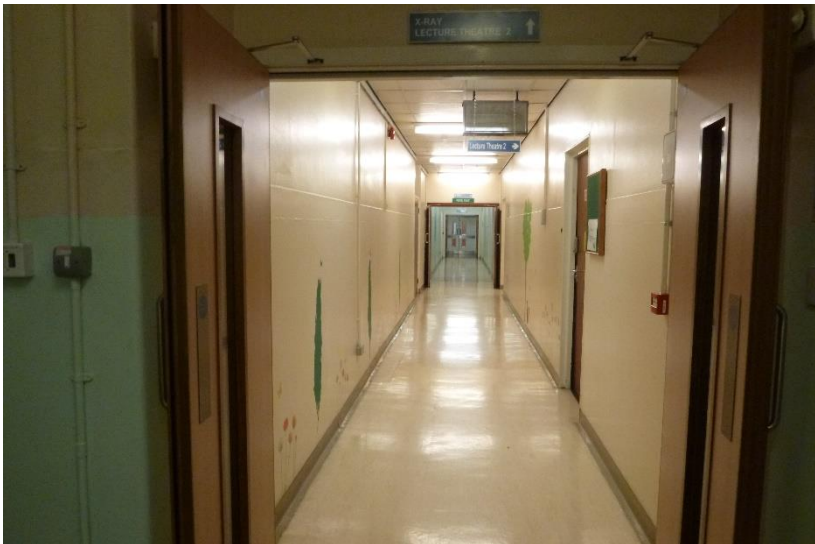
Figure 9: Modern lower-ground floor corridor; the original floor-plan is all but lost on this floor
