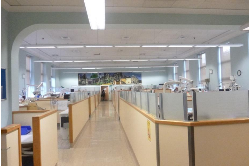
Figure 8: Double-height, second-floor clinic today. The sawtooth rooflights are concealed by the modern suspended ceiling
