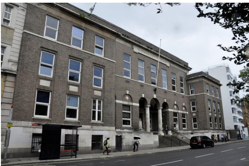
Figure 3: Front elevation of the former EDC
