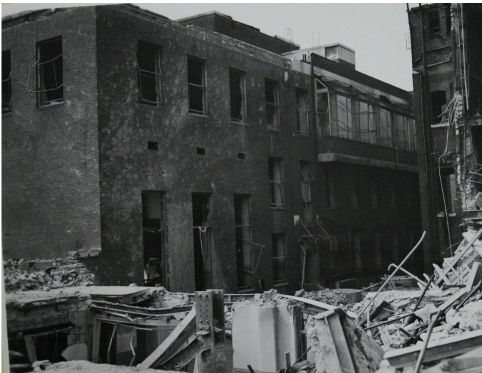
Figure 7: Bomb damage to the north wing in 1944, viewed from the north-east
