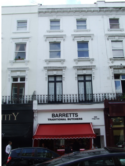
View of front of 40 Englands Lane.
