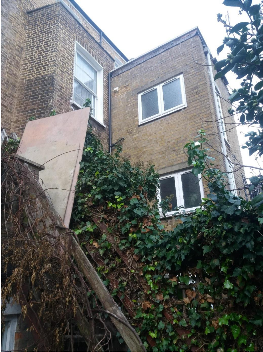
Figure 7 views of rear extension at no.72
