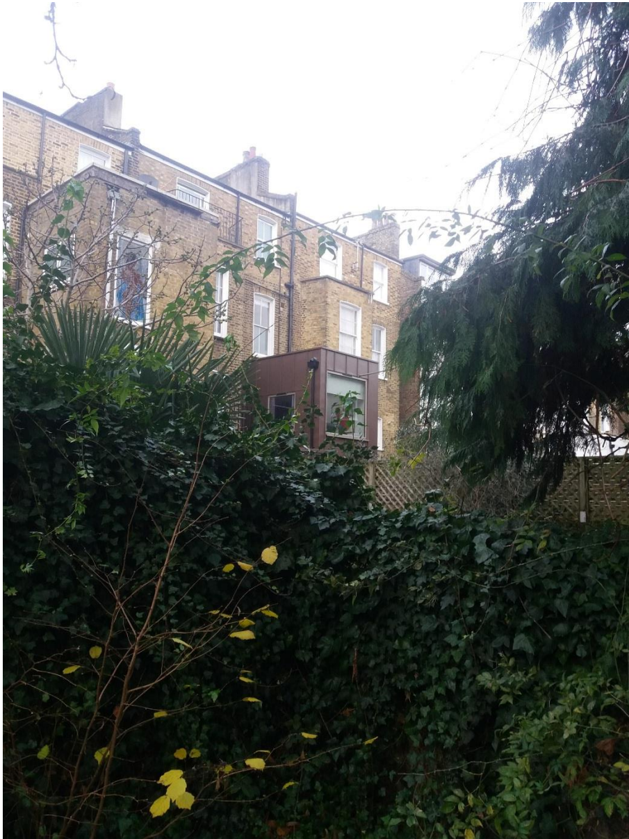
Figure 5 View of extension at no.78
