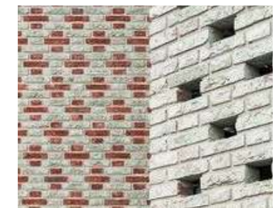
Patterns derived from existing brickwork.
