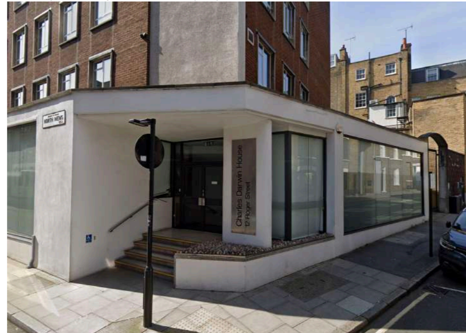
Existing entrance to reception with metal signage on column.
