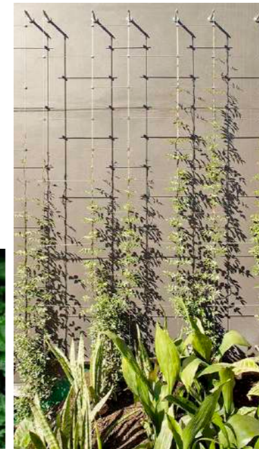
Wire rope plant trellis system.
