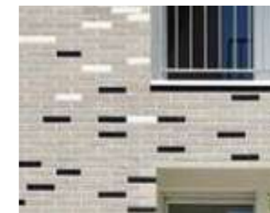
Glazed bricks within brickwork.
