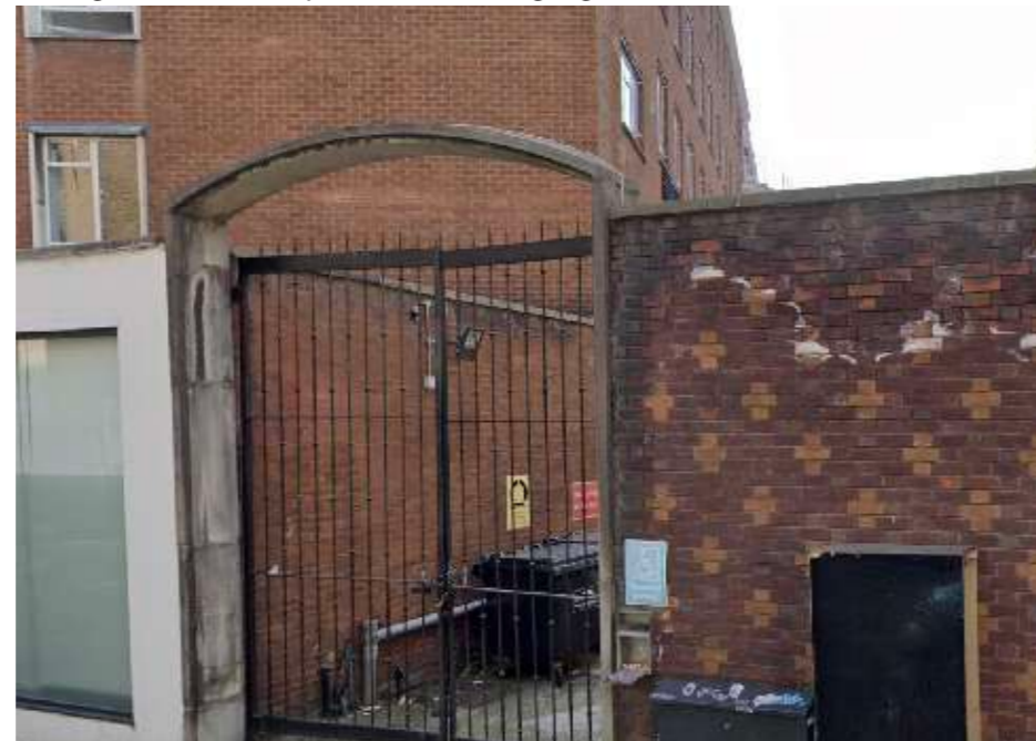
Existing gate into courtyard area.
