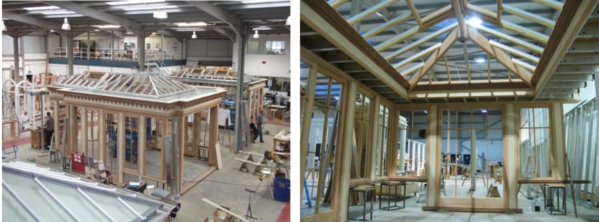
Fig. 9 & 10 – General Photos of Vale Garden Houses factory assembly hall
