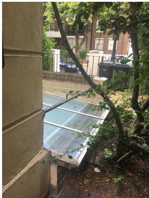
Existing roof light
