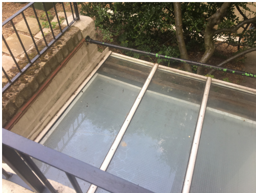
Existing roof light
