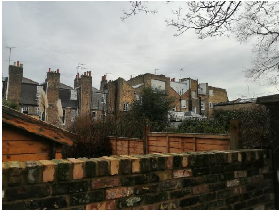
Photo 8: Extensions made to the rear of properties on Arlington Road
