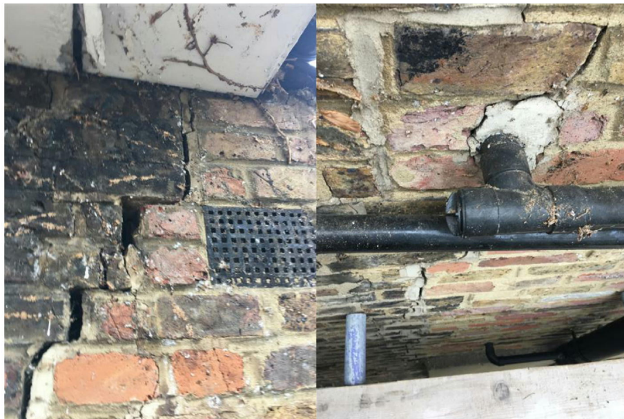
Separation between main building and outrigger
