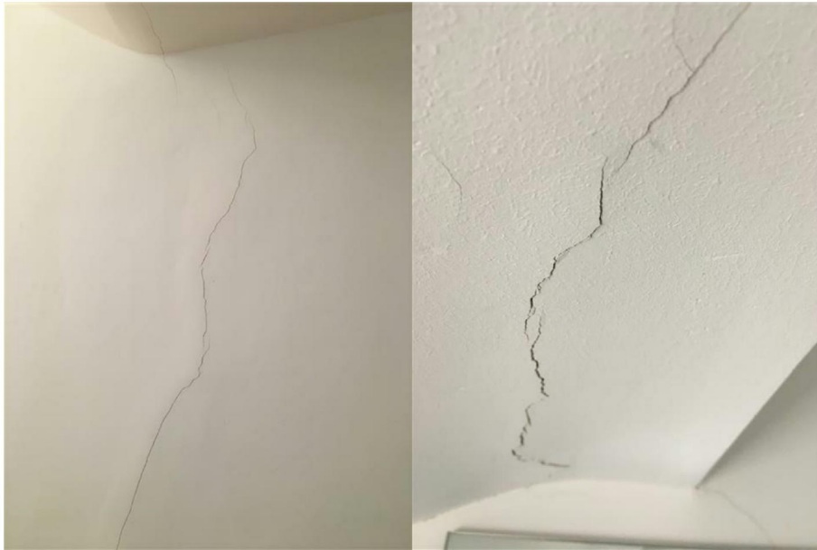
Fracturing at junction between main body and rear outrigger
