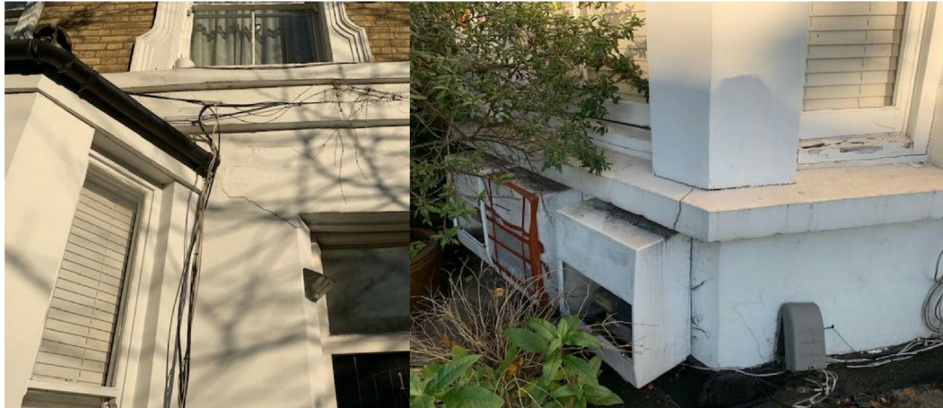
Cracking around front bay window
