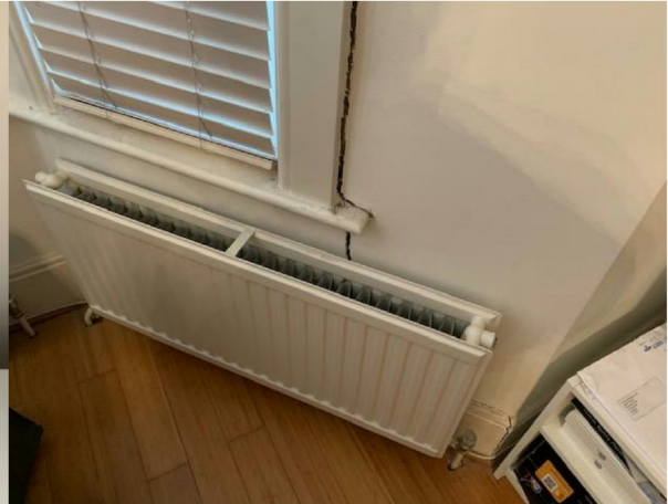
Cracking to front bay in Flat A
