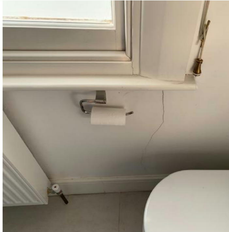
Cracking in en-suite to Flat C
