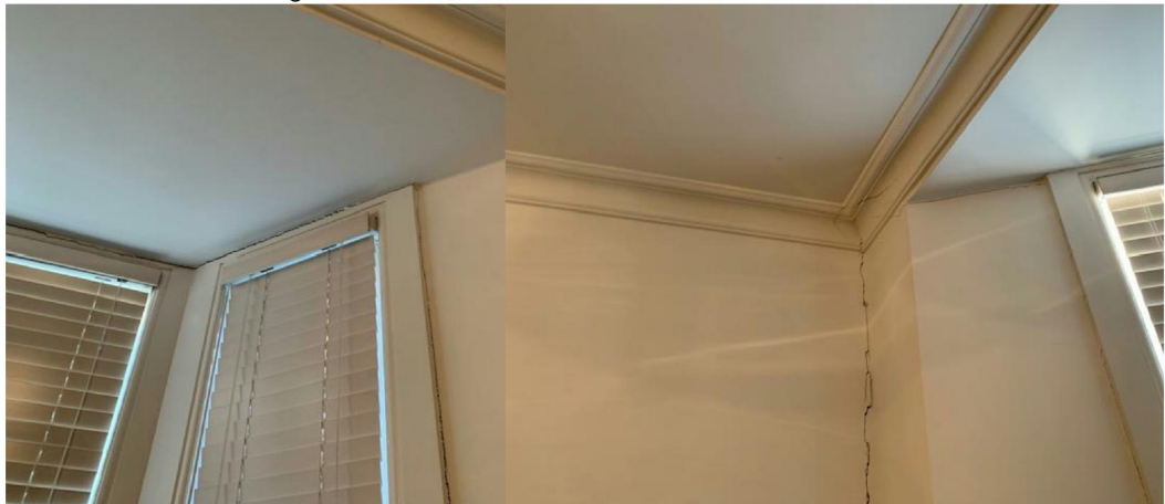
Front Wall cracking in Flat B
