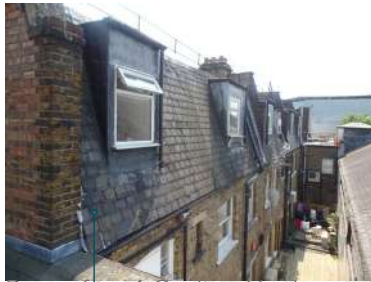
Rear of no.4 Grafton Yard
