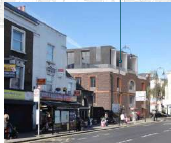
Proposed 187 Kentish Town Road with large size dormer & residential with different roof eaves and ridge heights to roof space
