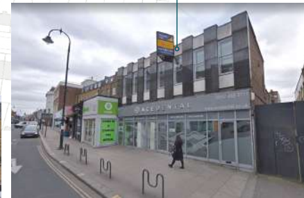
158: Office & dental Service building, with Stone & tile finished to its first floor
