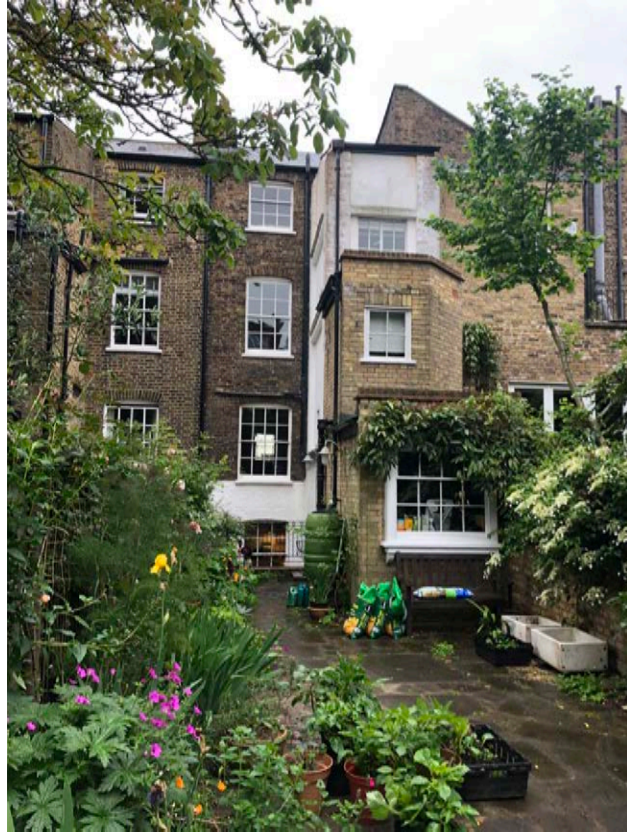
27 Downshire Hill - existing rear extension
