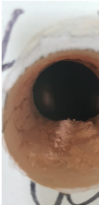
Photograph 2 – Wall 1 two leaf terracotta hollow pot with void between
