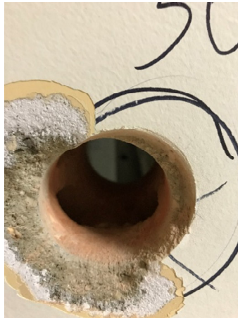
Photograph 33 – Wall 30 blockwork (filled in door)
