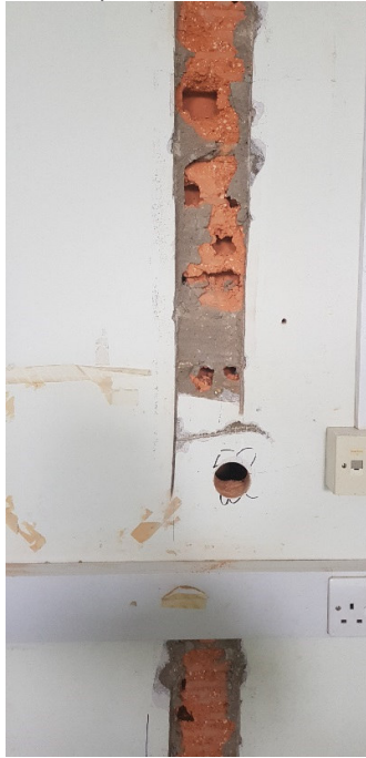
Photograph 1 – Wall 1 two leaf terracotta hollow pot with void between
