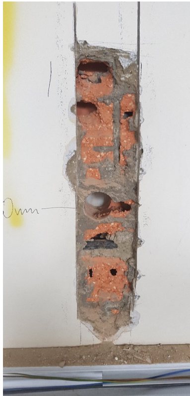
Photograph 4 – Wall 3 250mm masonry wall (Taken inside room 221)
