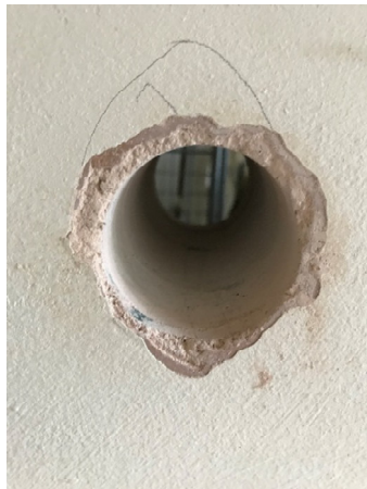
Photograph 33 – Wall 30 blockwork (filled in door)
