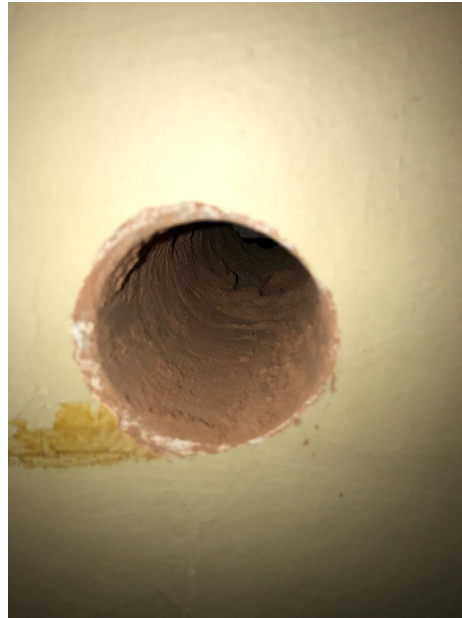
Photograph 5 – Wall 3 250mm masonry wall (Taken inside cold room 214). Refer to photographs 36-38 for more details
