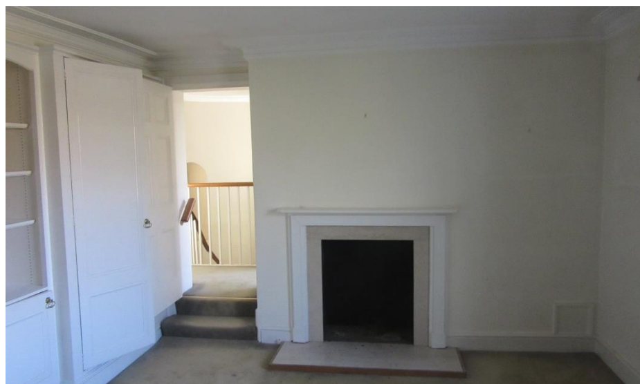
Figure 26: First floor front room, depicting mid-20 th century fire surround and modern fittings (left); the skirting and cornicing are modern inappropriate additions. The change in level to the carriageway extension is clear.
