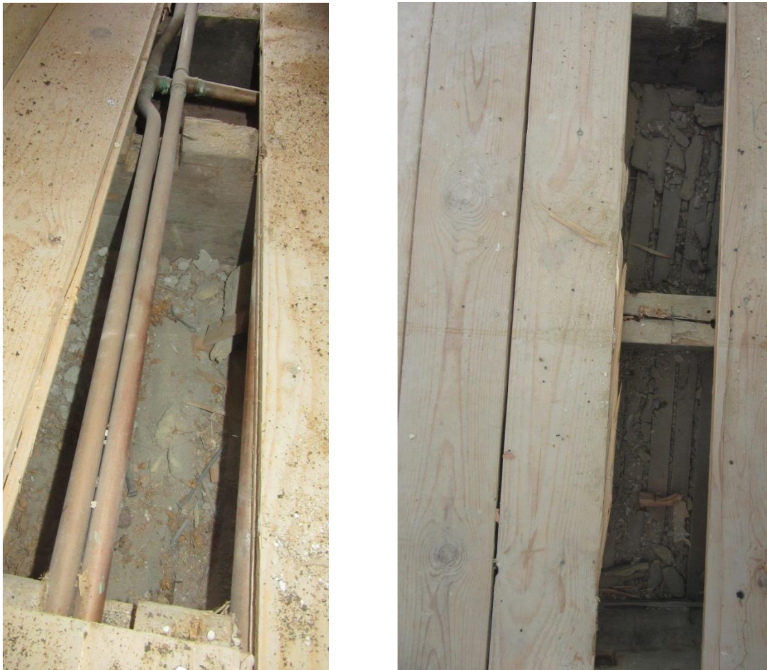
Figure 27: The floor structure of the first floor (over-carriageway extension left, rear room right), indicating original joists and ceiling structure topped by modern boards.
