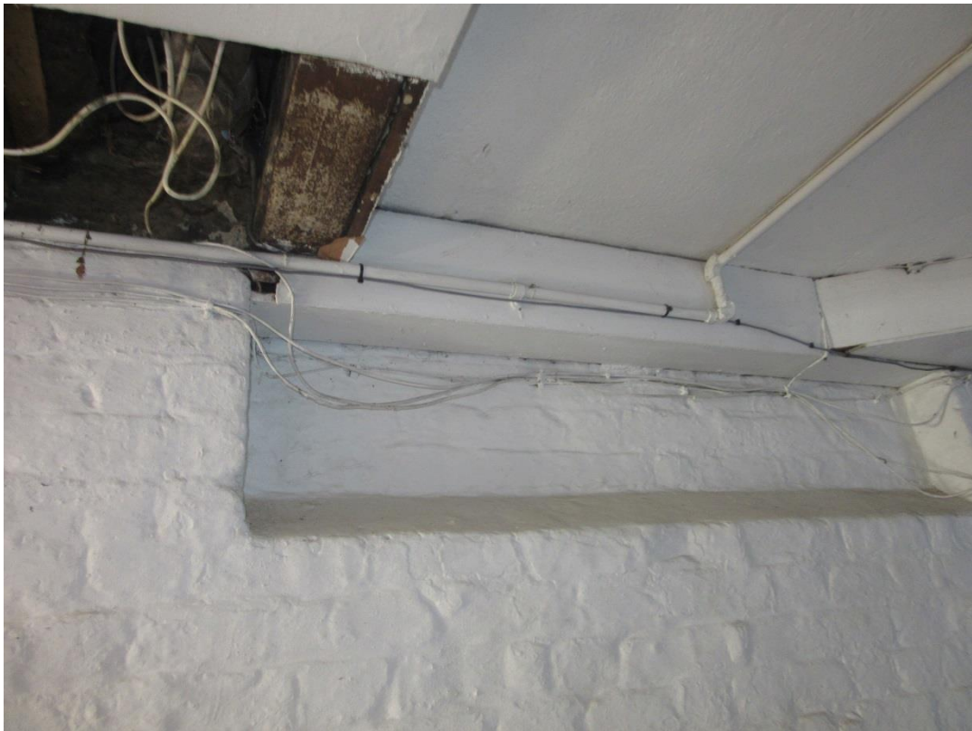
Figure 20: Historic blocked window opening and iron beam within the former carriageway, now more of a pedestrian passageway.
