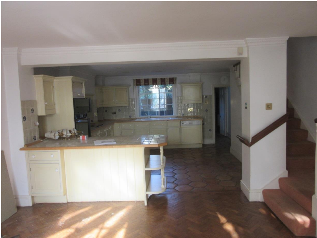
Figure 18: Lower ground floor looking towards the front room, illustrating 1950s staircase (altered 1988) with 1950s nibs and downstand (RSJ) outlining the original spine wall.
