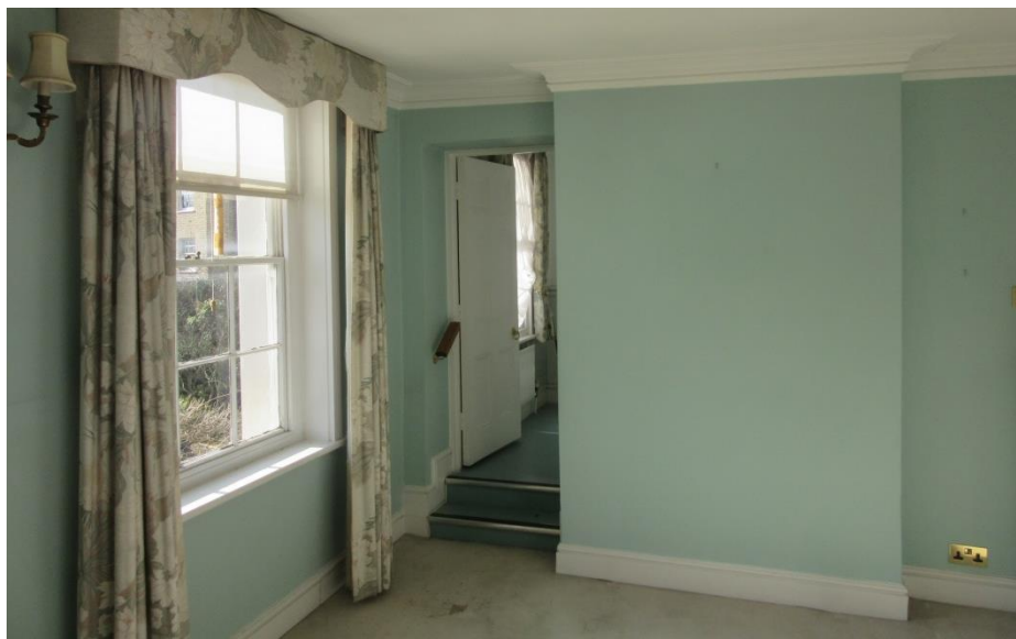
Figure 25: First floor rear room, depicting blocked fireplace, inappropriate 20 th century architectural detailing, and 1980s doorway made into adjoining shower room.
