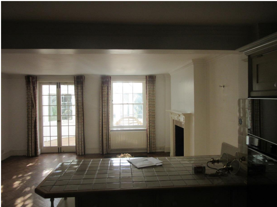
Figure 19: Lower ground floor looking towards the rear room, illustrating inappropriate fire surround brought in in 1988 and 1980s French doors leading into the 1980s conservatory.
