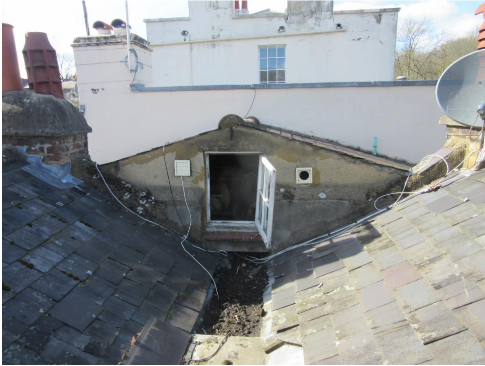
Figure 28: The original two pitches of the M-roof structure with central valley gutter, with the unusual and uncomfortable latter pitched roof above the carriageway extension.
